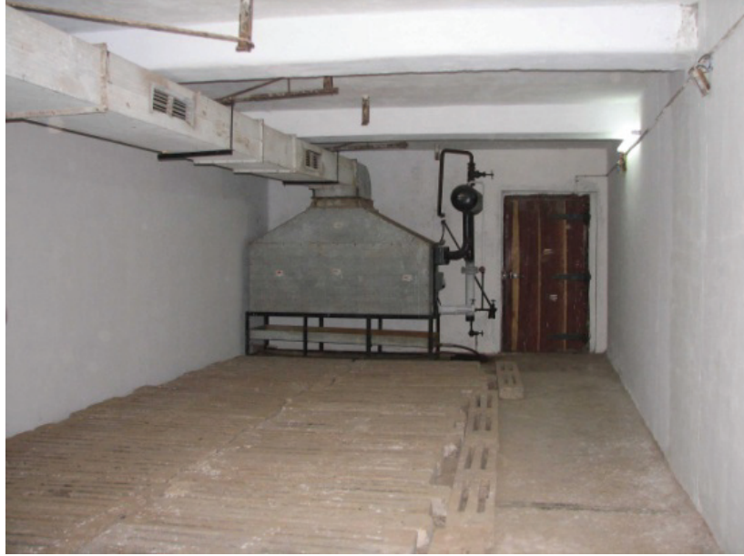
Figure 3. 7: The commercial cold store in the city of Coimbatore. An ammonia evaporator sits at the back of the room, and cool air is circulated through a large duct at the top of the room.
