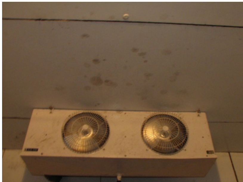
Figure 4. 37: Mould on the ceiling next to the evaporator in the experimental cold store.
