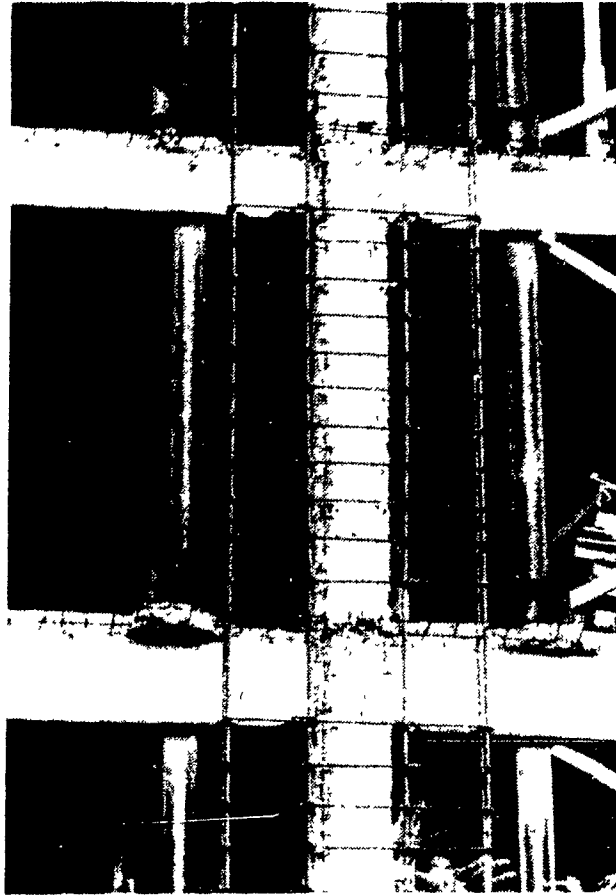
Figure 3.18 Typical Enlarged Edge Column.
