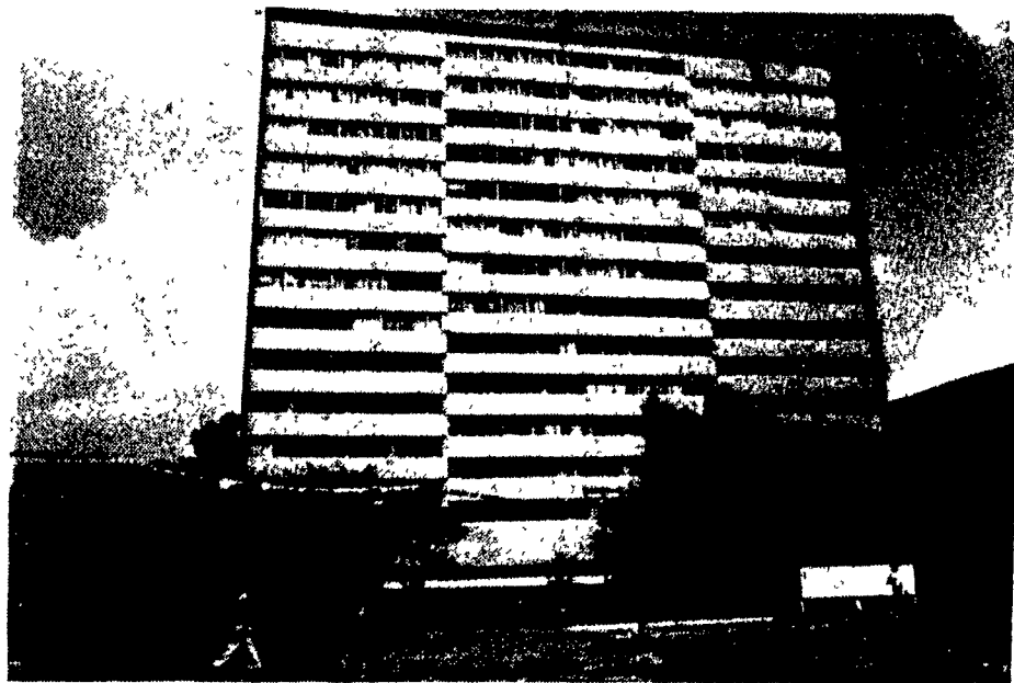
Figure 3.28 Fourteen Storey Apartment Building with Offset Floors which was Damaged in the 1985 Earthquake (Mitchell et al 1986).
