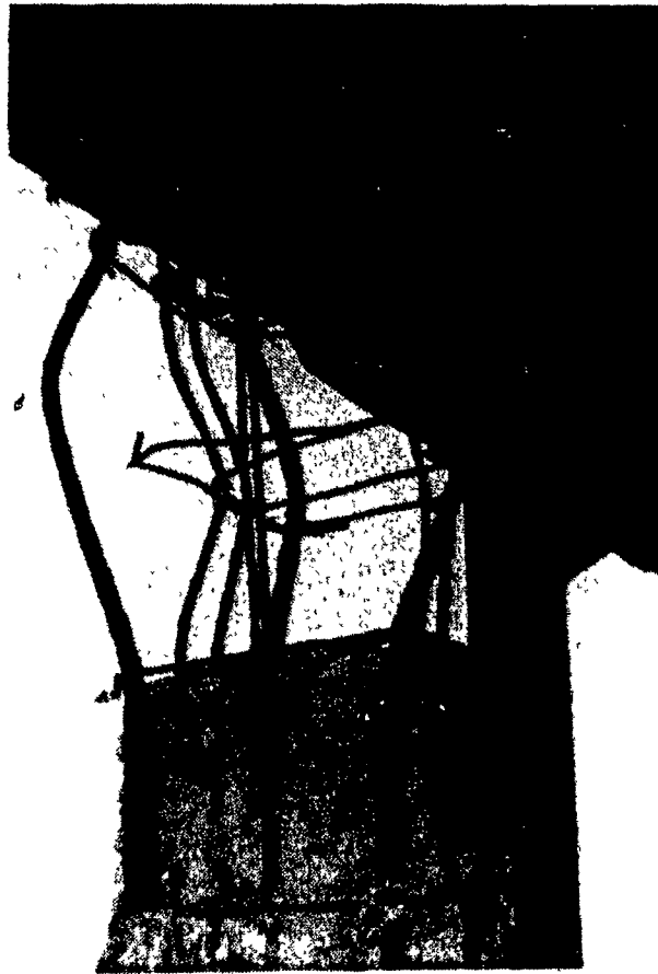
Figure 3.10 Shear Failure of a Fourth Floor Exterior Column 26 .
