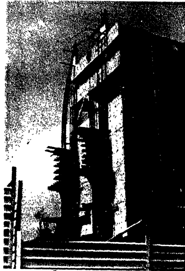
Figure 3.30 Construction of End Shear Walls.
