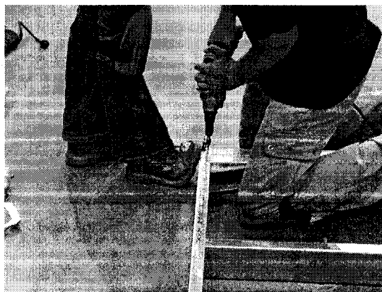
Figure 3.9: Back-to-back chord stud and bottom track connection with framing screw and framing screw gun
