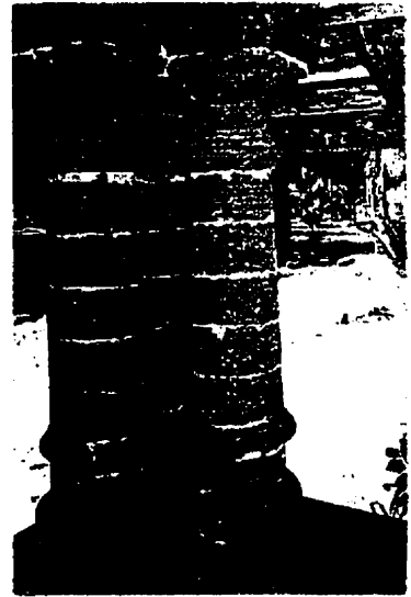
Picture 3.31: Masonry pillar built of cut laterite.
