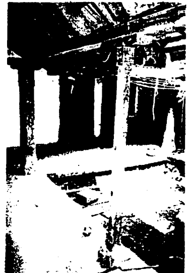
Picture 3.16: Wall plate supported on pillars around the courtyard.
