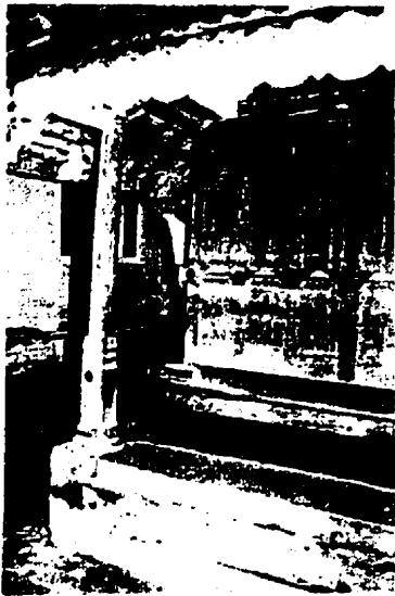
Picture 3.8: Shows the corner detail of plinth level beam over which 'nira' is erected.
