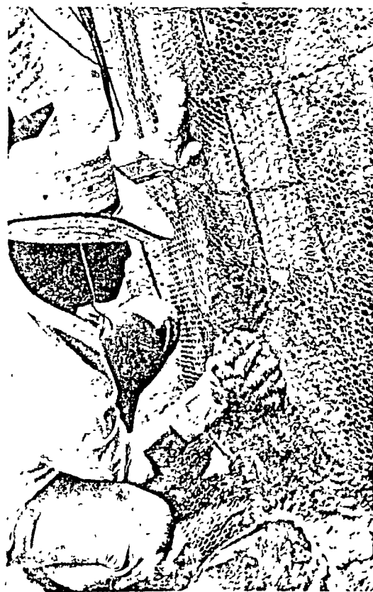
Fig. 7.24 Mortar plastering. (National Academy of Sciences)
