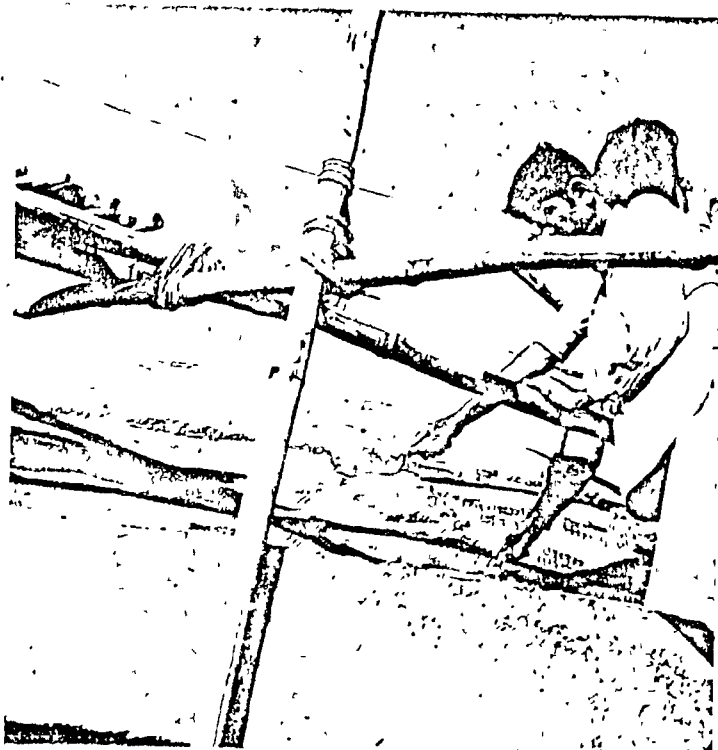
Fig. 7.33 Placing of mortar. (Ferro- cement Journal)
