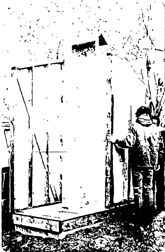
Fig. 11.11 Assembly of solar heated and sulfur impregnated toilet house.
