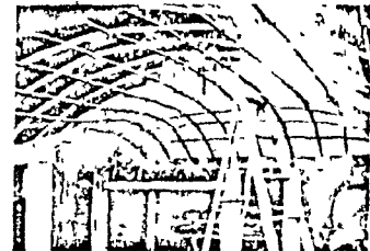
Fig. 7.9 Burlap over the lattice work.
