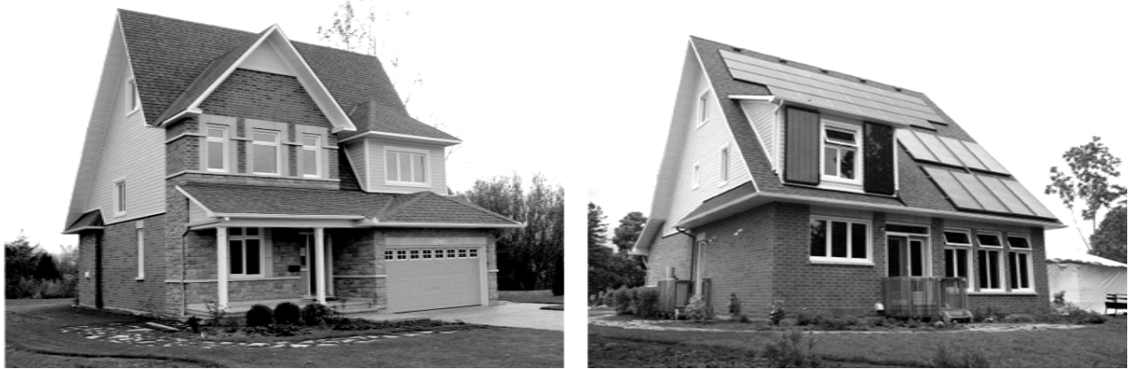
Figure 4.2 – Minto’s EcoHome – the rear roof features “solar water collectors” and “photovoltaic solar electricity panels” source: Minto Group Inc. 2008
