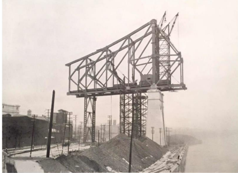
Stage II: Progress on North Main Span
