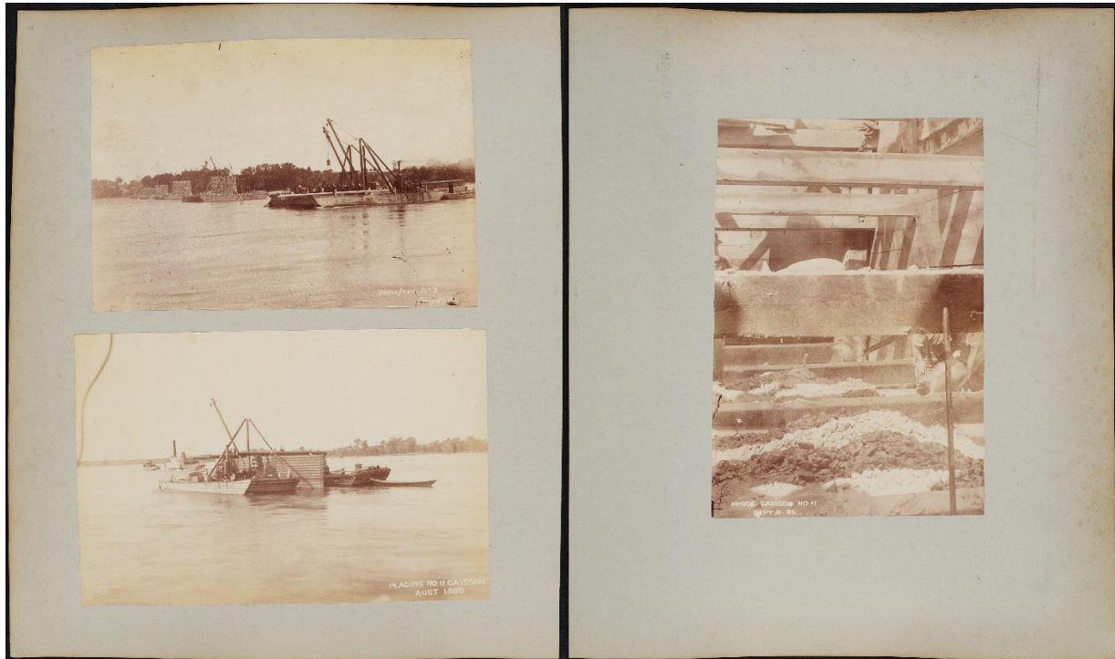
Figure 4.12: Top left: View from No. 9 , July 21, 1886. Bottom left: Placing No. 11 Caisson , August, 1886. Right: Inside Caisson No. 11 , September 11, 1886 [LAC: C-256 Accession 1987-161, Box 2 #4, pages 13 and 14].
