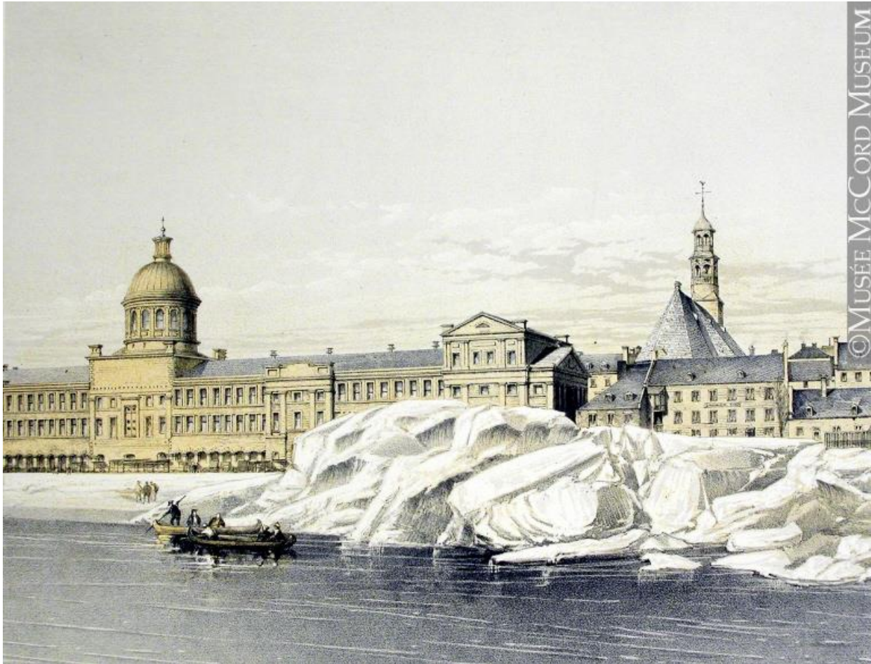
Figure 2.5: Shoving of ice upon wharves in front of Montreal , Anonymous, Construction of the Great Victoria Bridge , 1860. [MM: M15934.18].
