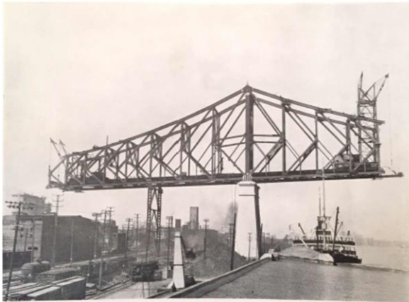
Stage III: Concurrent Erection of North Anchor and Cantilever Arm
