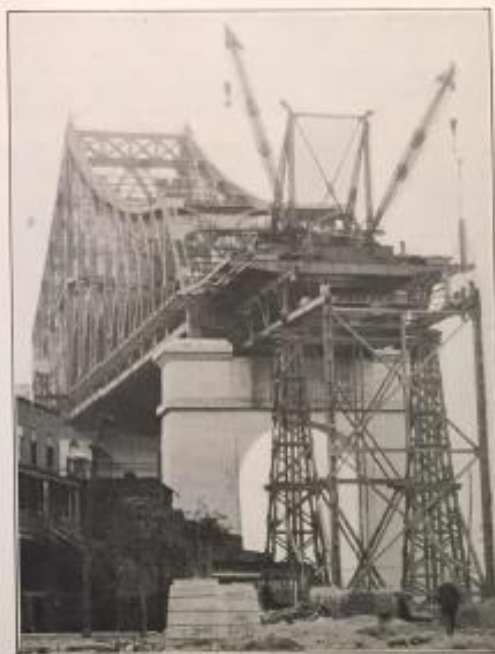
Figure No. 23.—North Approach—Typical Method of Erection—Second Stage.
