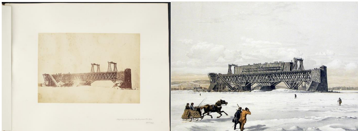
Figure 3.9: (Left) Staging for the centre tube , William Notman, 1859 [LAC: Alex Ross Album]. (Right) Centre Tube in Progress—From the Ice , Kell Brothers, 1860 [MM: M1593.27].
