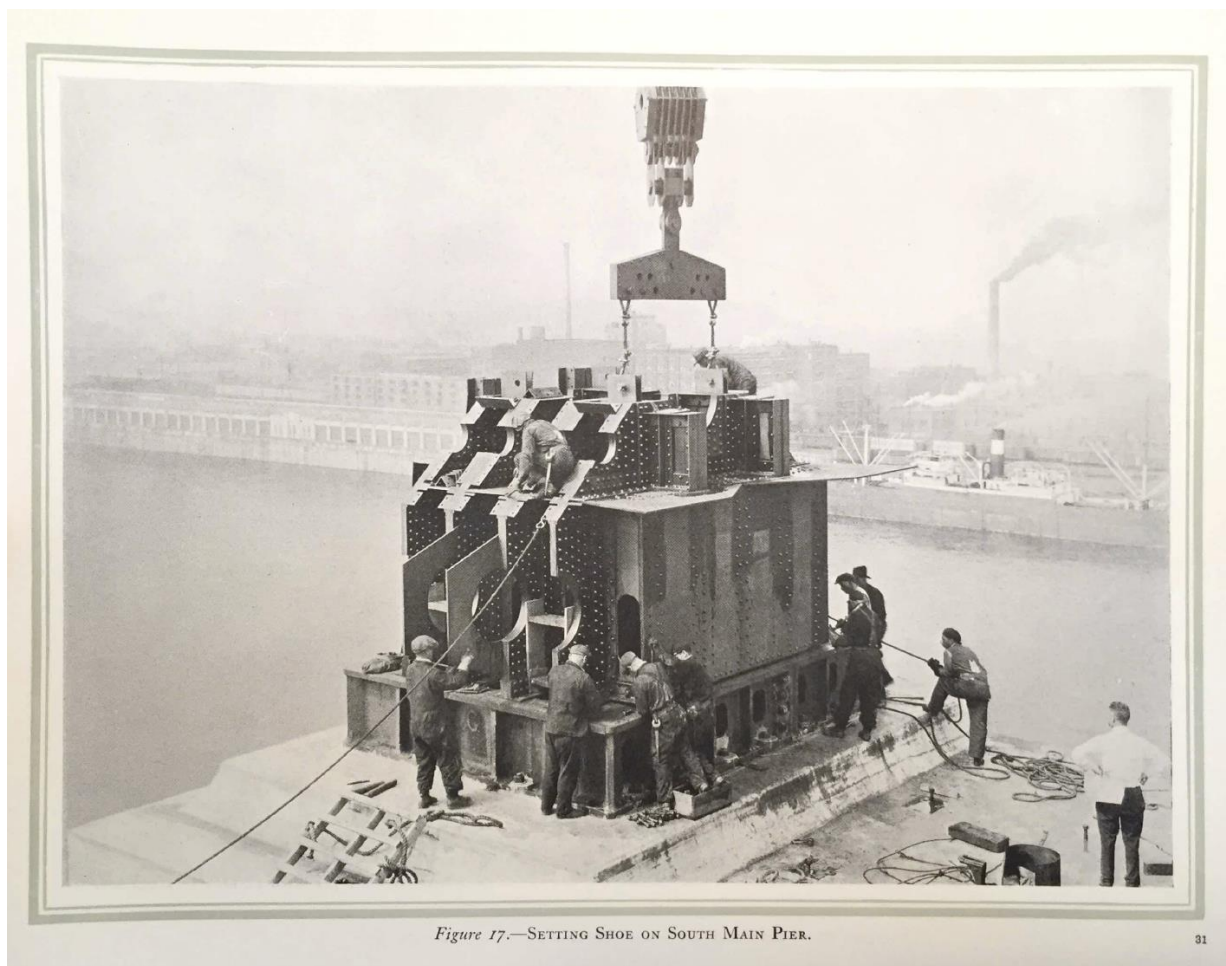
Figure 4.25: Setting Shoe on South Main Pier
