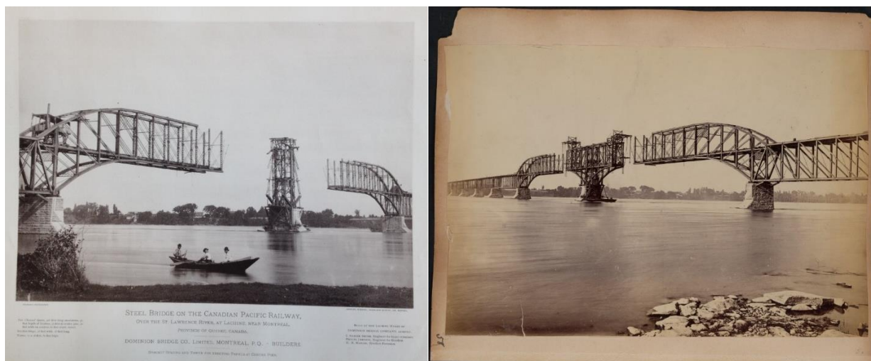
Figure 1.5: Left: Steel Bridge on the Canadian Pacific Railway: Centre Staging , Alexander Henderson [LAC: 1976.72 SC 0027 PA-117233]; Right: Cantilever from the South Shore [LAC: C-256 Accession 1987-161, Box 2 #3, Image 58].
