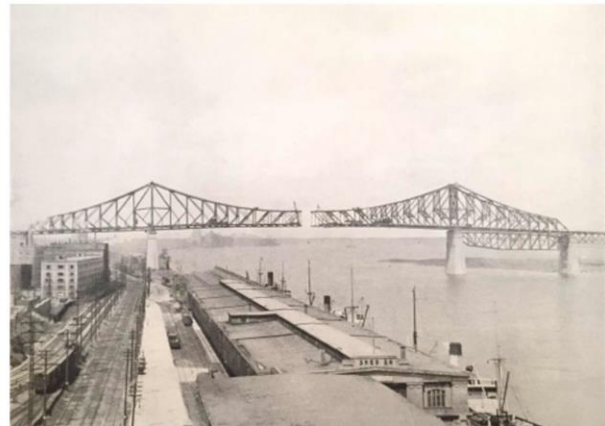
Stage IV: Progress on Main Span
