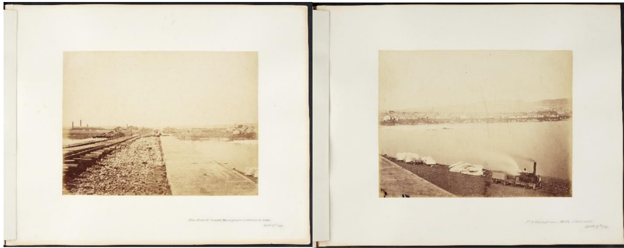
Figure 4.0: No. 1 Grand Trunk Works from Entrance to Tube and No. 2 View from North Abutment, William Notman, April 19, 1859 [LAC: Alex Ross Album].
