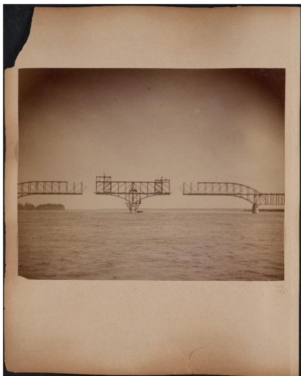
Figure 3.25: The final image in the scrapbook showing the superstructure. [LAC: C-256 Accession 1987-161, Box 2 #3].
