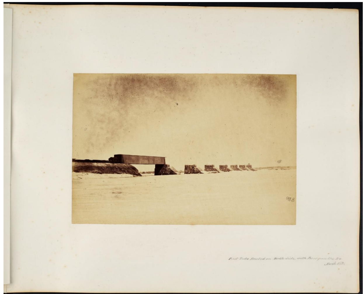
Figure 4.5: First Tube Erected on North Side, with Piers from the Ice , William Notman, March 1858 [LAC: Alex Ross Album].
