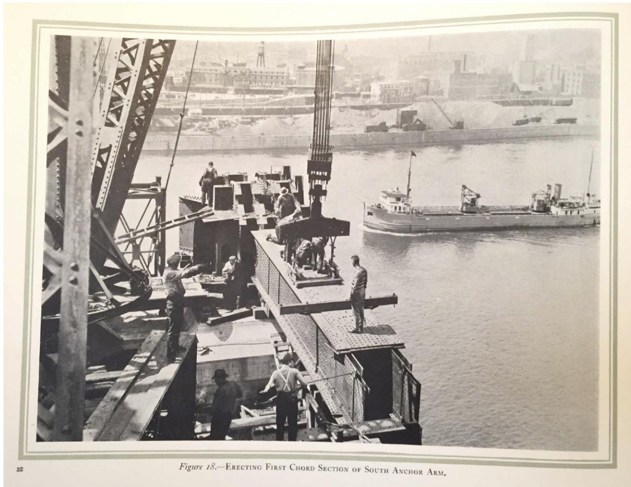
Figure 3.31: Image showing advances on the bridge with the busy port in the background. [DBC, Superstructure of Montreal Harbour Bridge, 22 (Figure 18)].
