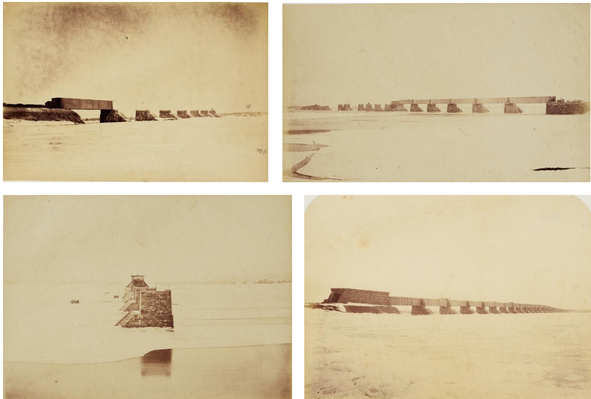
Figure 4.9: Upper Left: First-Tube Erected on North Side, with Piers from the Ice, March 1858. Upper Right, Bridge in Progress from Point St. Charles, Dec. 18th, 1858. Lower Left: Pier No. 12 Looking In, March 1859. Lower Right, General View of the Bridge Completed, January 1860 [LAC: Alex Ross Album].
