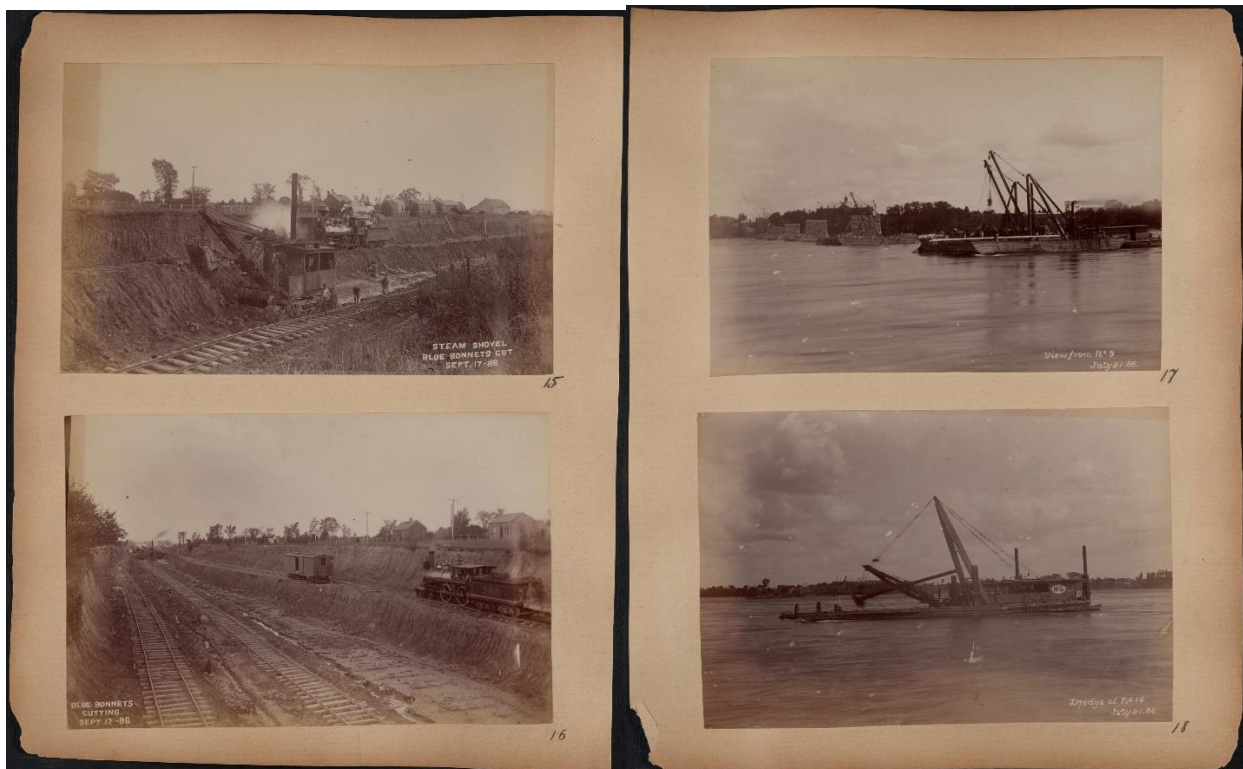
Figure 3.22: Left: Cut and Fill operations , Right: Cofferdams . [LAC: C-256 Accession 1987-161, Box 2 #3, Photographs fifteen to eighteen].
