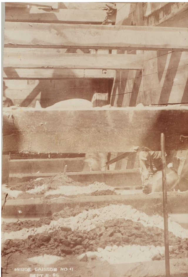
Figure 4.17: Inside Caisson No. 11, Sept 11-86 [LAC: C-256 Accession 1987-161, Box 2 #4, page 14].
