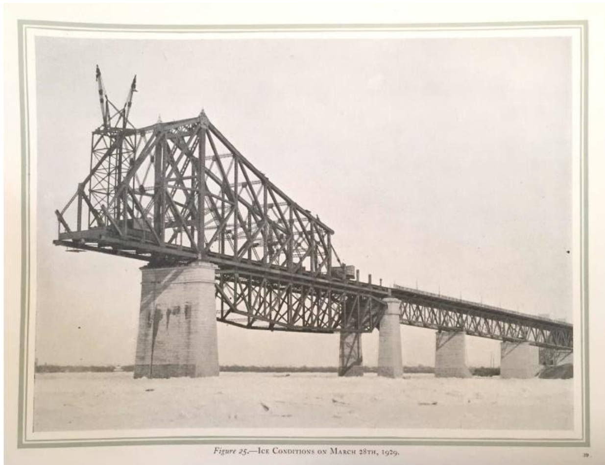
Figure 4.7: Ice Conditions on March 28th, 1929 [Bridge [DBC, Superstructure of Montreal Harbour Bridge, 39 (Figure 25)].
