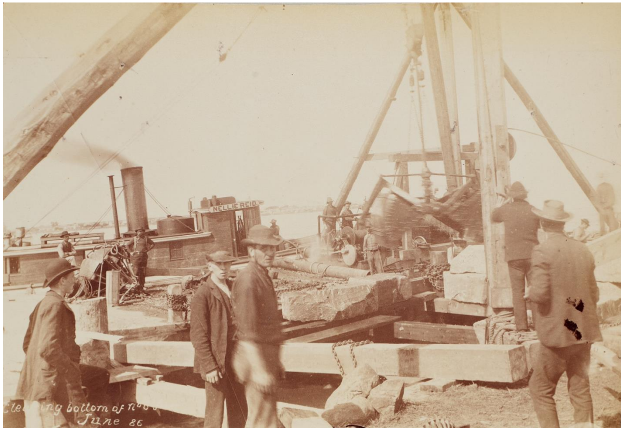
Figure 4.16: Clearing the Bottom of No. 6 Pier, June 1886 [LAC: C-256 Accession 1987-161, Box 2 #4, page 10].
