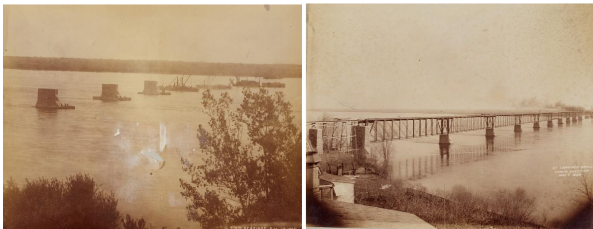
Figure 4.11: Left: View of Bridge, August 2, 1886 , and, Right: St. Lawrence Bridge during Erection, May 5, 1887 [LAC: C-256 Accession 1987-161, Box 2 #4, pages 1 and 44].
