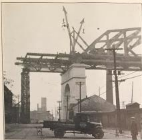
Figure No. 22.—North Approach—Typical Method of Erection—First Stage.
