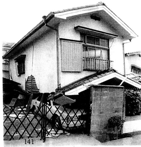
Fig.1.10 Collapse by Earthquake in 1993, Kobe (Matumura, 1996)
