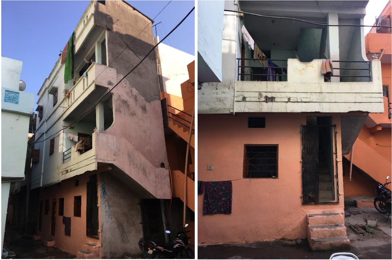
Fig 5.19: Residence B01- exteriors.
