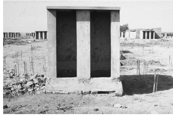
Fig. 3.38: Service core construction
