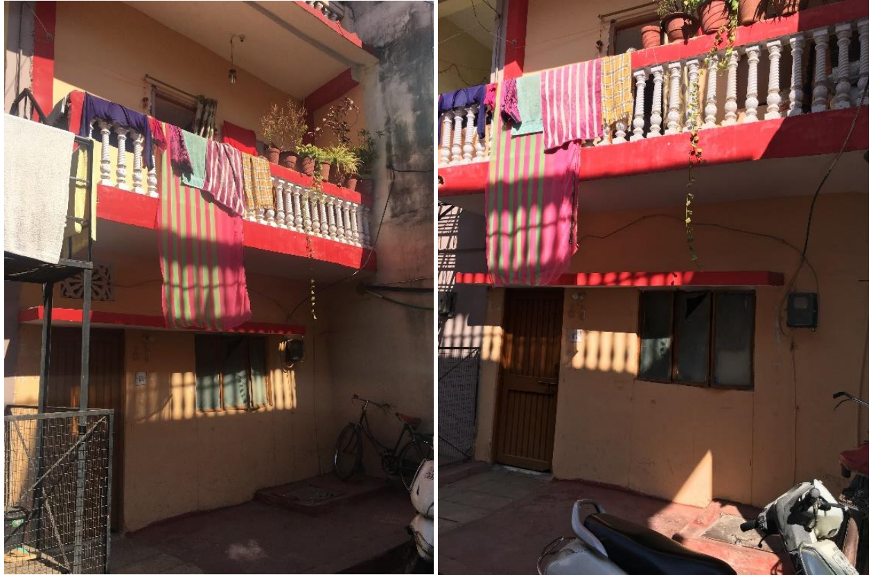
Fig 5.22: Residence B02- exteriors.
