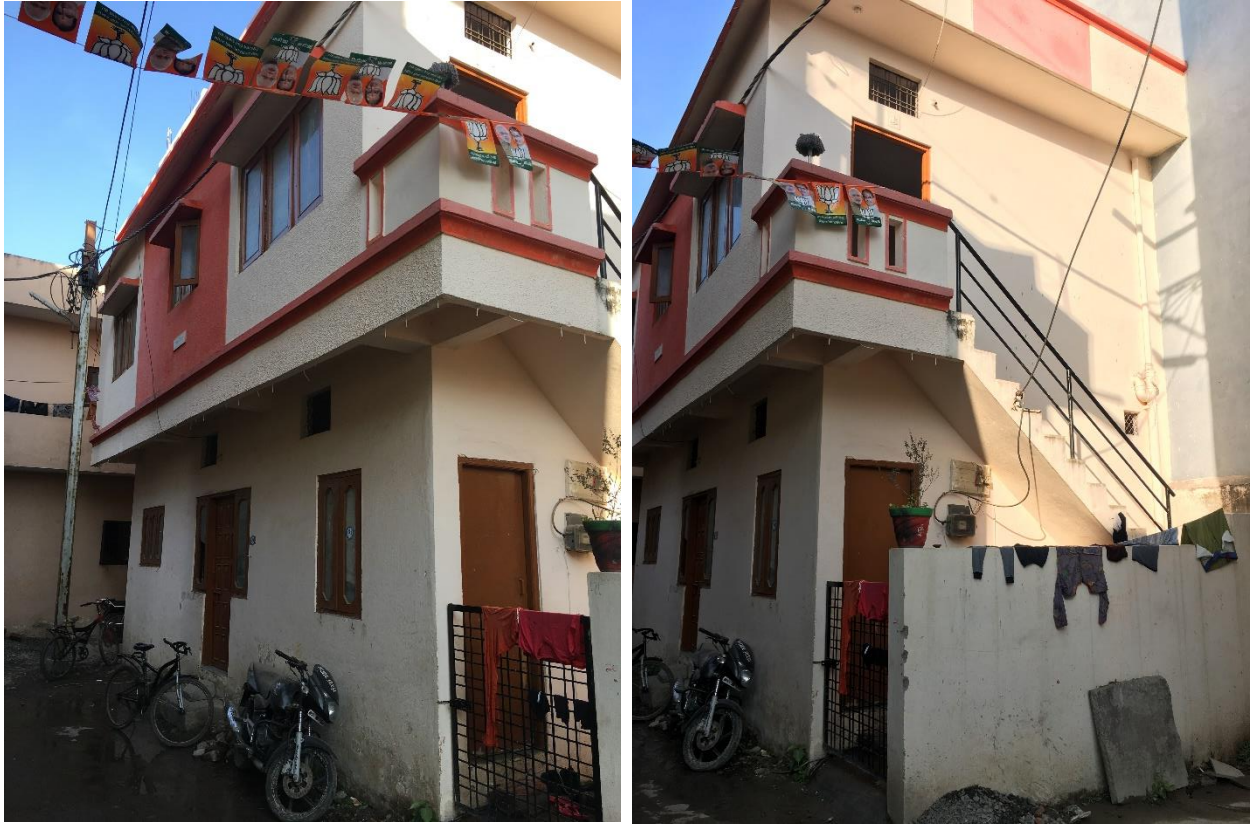
Fig: 5.25: Residence B03- exteriors.
