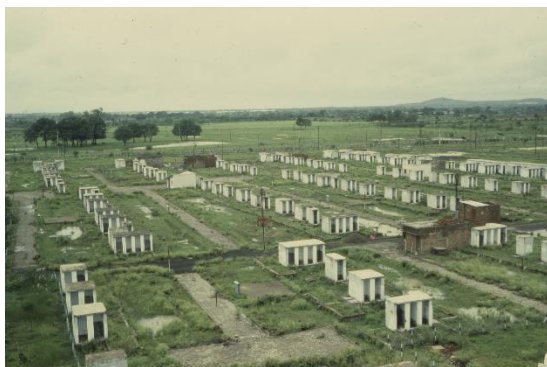
Fig. 3.40: Construction of Aranya
