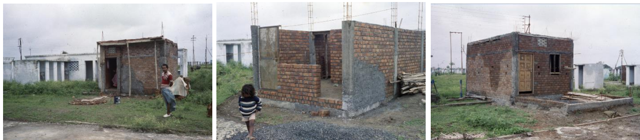
Fig. 4.7: Construction of houses at Aranya
