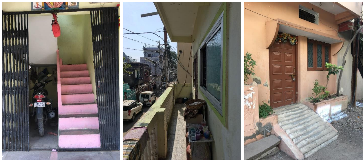
Fig 5.32: Residence B06- access stairs, balcony and main entrance to ground floor residence.
