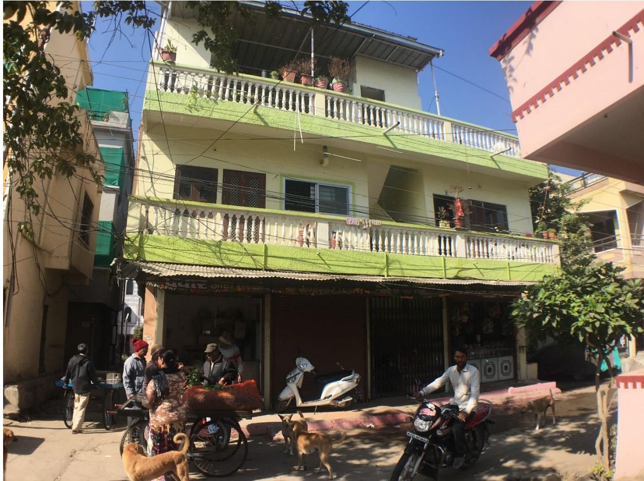
Fig 5.33: Residence B06- exterior.
