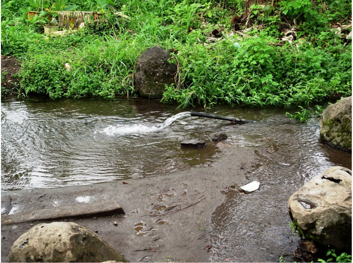
Photo 2: Pipe above is used by residents around source to fill up buckets. Pipe from spring to the supply tank is underwater from right to left.
