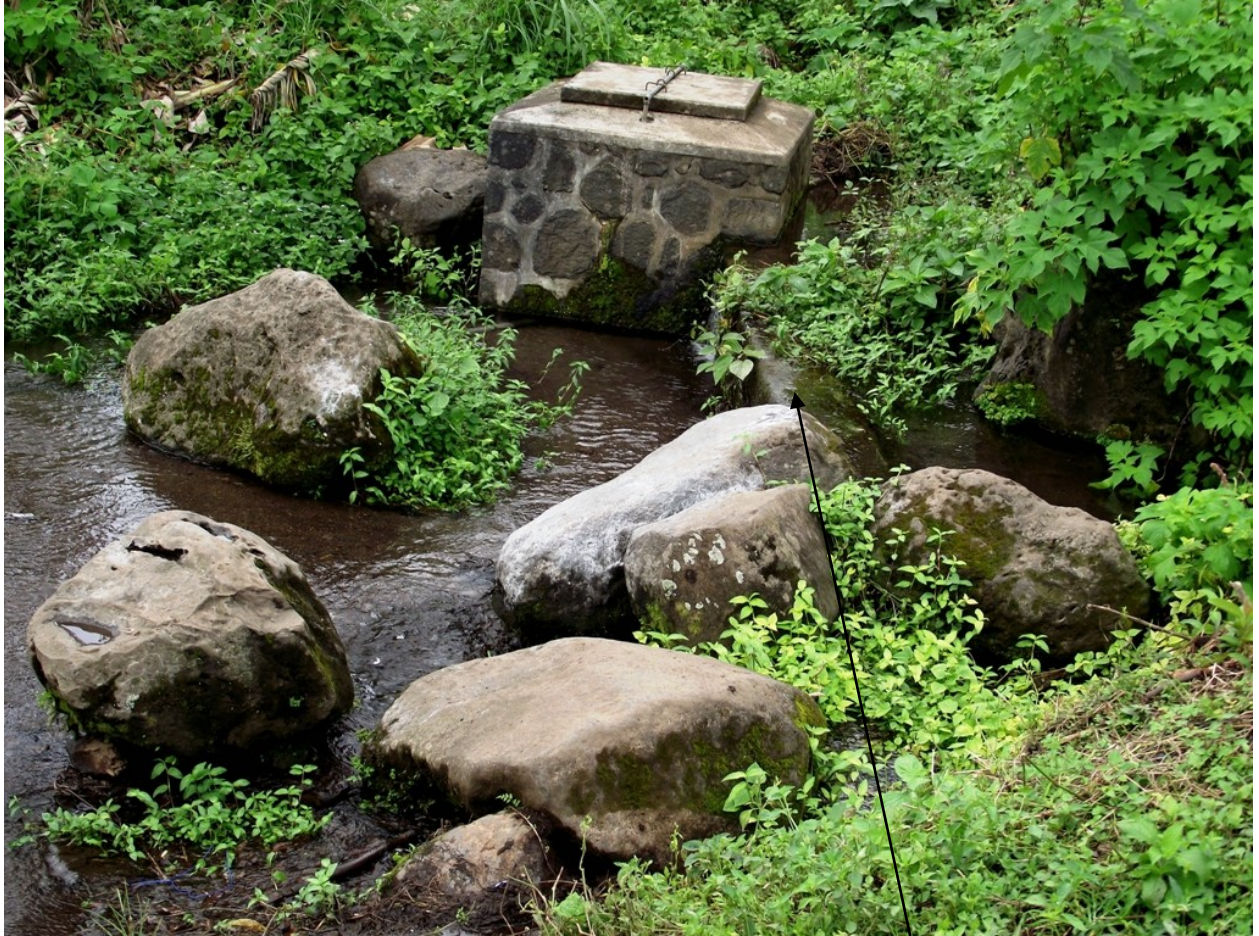
Photo 3: Spring emerges from the right side and there is a small dam and weir. The pipe to the supply tank harnesses water from that area. There is a lot of excess capacity that is not harnessed that flows out as a stream
