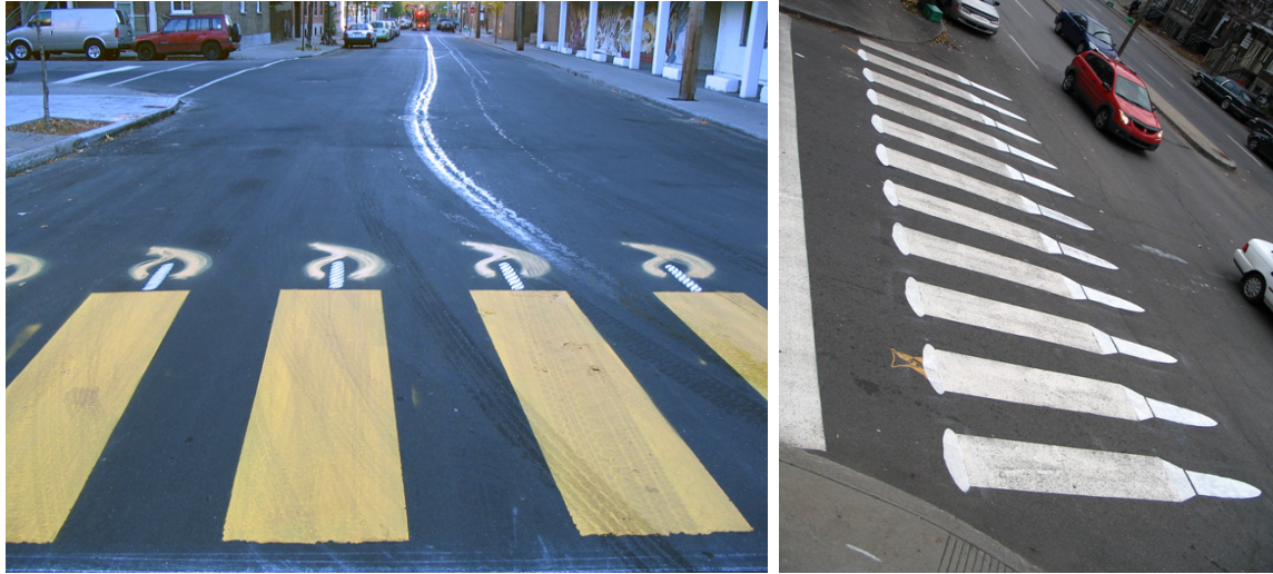
Figure 9 Candles , Fairmount Ave and Saint-Dominique St, September 2004 and Full Asphalt Jacket , Rivard St. and Saint-Denis Blvd., Montreal, Quebec. October 2004.
