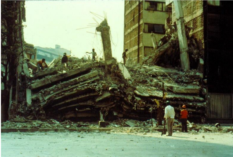
Fig 2.1. Progressive collapse of 9-storey flat plate structure in the Mexico City earthquake of 1985 (Mitchell et al. 1986)
