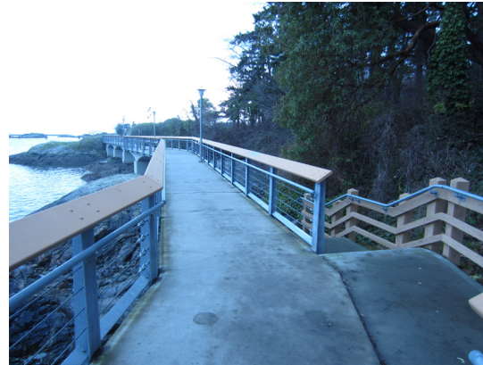
Figure 29: The intertidal zone access stairs nearest to Barnard Park.
