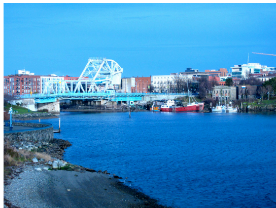
Figure 21: Another potential view to frame, this one would be of the new Johnson Street Bridge.
