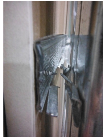
Figure 3.16 Close up of a damaged resilient channel
