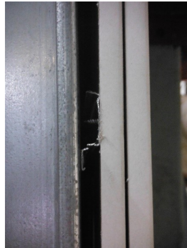
Figure 2.23 Double layer gypsum fastened to the resilient channels
