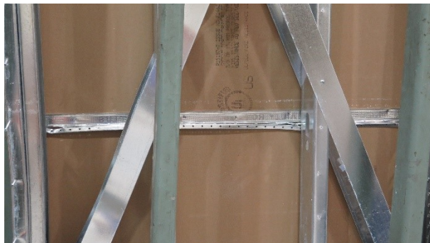
Figure 3.15 Damaged resilient channel
