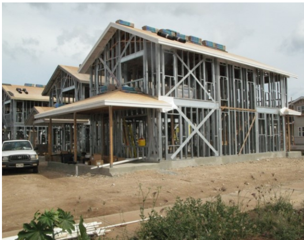
Figure 1.1 Cold-formed steel building with strap-bracing
