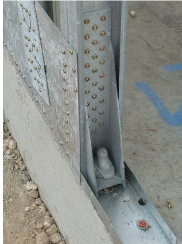
Figure 1.3 Hold-down device screw connected to the frame and anchored to the foundation
