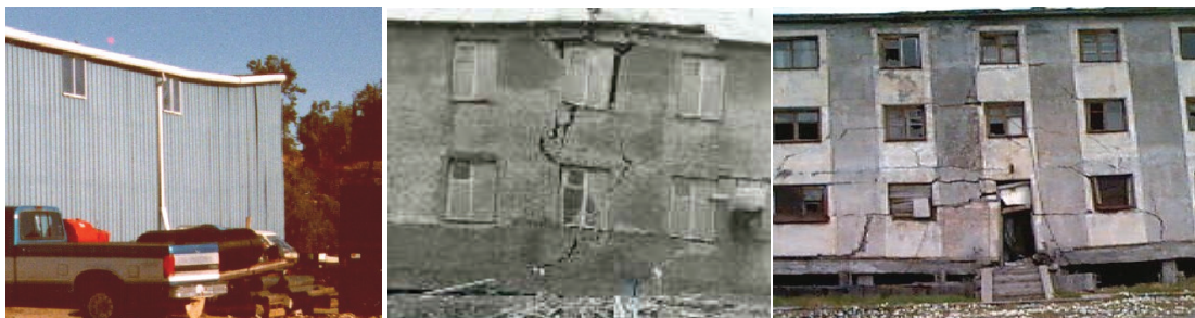
Figure 9.11 Examples of buildings destroyed by melting permafrost. Apparent uplift of the right side of building due to frost heaving (left – GSC, 2006). Differential settlement followed by extreme cracking of buildings (centre and right - Brouchkov and Himenkov, 2006).
