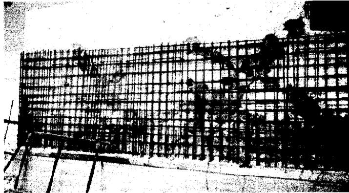
Figure 4-4: Shear walls repaired by concrete jacking (Elenas et al., 2002).
