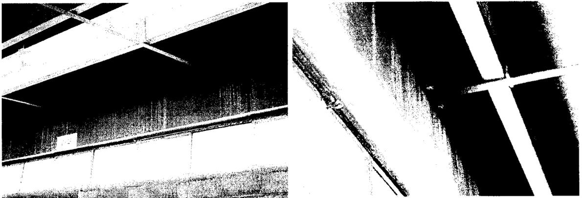
**Figure 2-11: Steel straps installed previously to minimize out-of-plane bowing of the perimeter wall.**
