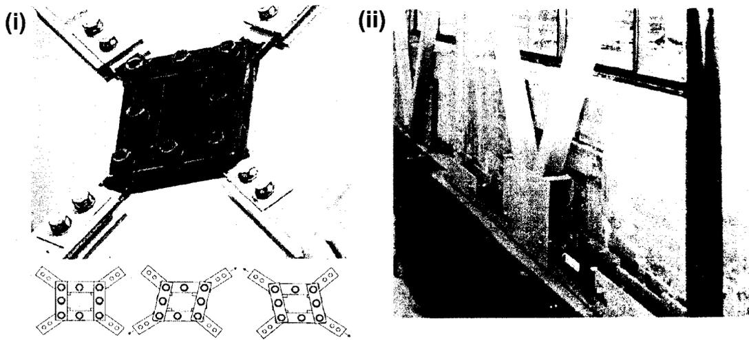
Figure 4-6: Steel brace retrofit incorporating: (i) a friction damper composed of clamped steel plates; (ii) viscous dampers (Foo et al., 2001).
