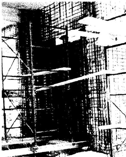
Figure 4-1: Adding a shear wall within an existing concrete frame (Elenas et al., 2002).
