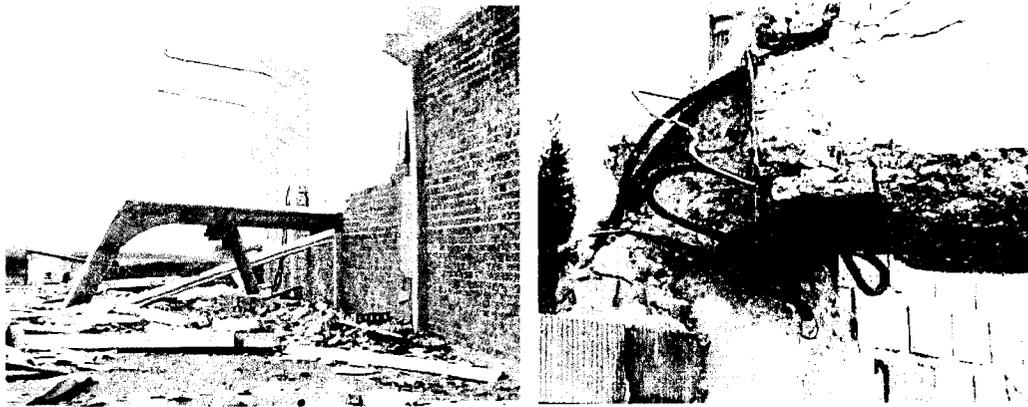
Figure 1-4: Shear failure of columns due to the influence of masonry-infilled walls (Saatcioglu et al., 2001).
