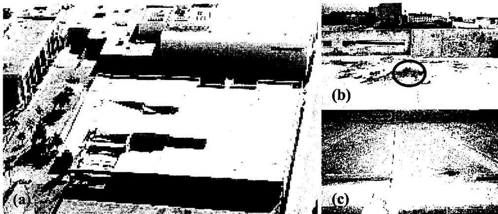
Figure 1-6: Failures of precast concrete diaphragms during the 1994 Northridge earthquake: (a) partial collapse of roof diaphragm; (b) buckling of chord reinforcement; (c) diaphragm cracks along the columns lines (Hawkins et al., 2000).
