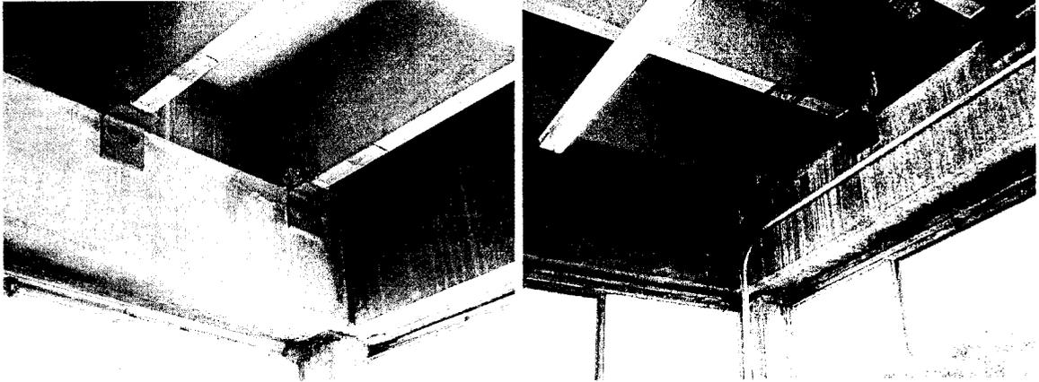
**Figure 2-10: Shear cracks at the double-tee supported ends.**
