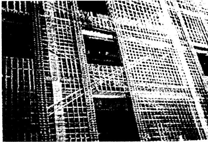
Figure 4-3: Addition of coupled shear walls outside a structure (Miller & Reaveley, 1996).
