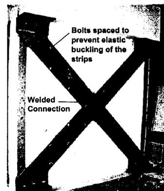
Figure 4-9: Masonry wall retrofitted using bolted steel strips (Taghdi et al., 1998).
