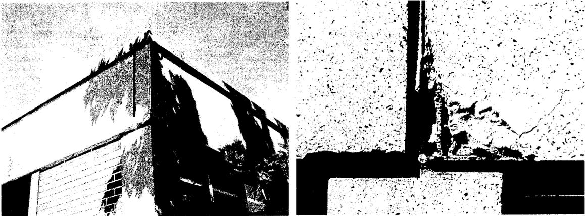
**Figure 2-8: Exterior condition of the building and deterioration at an exterior beam-to-column support.**
