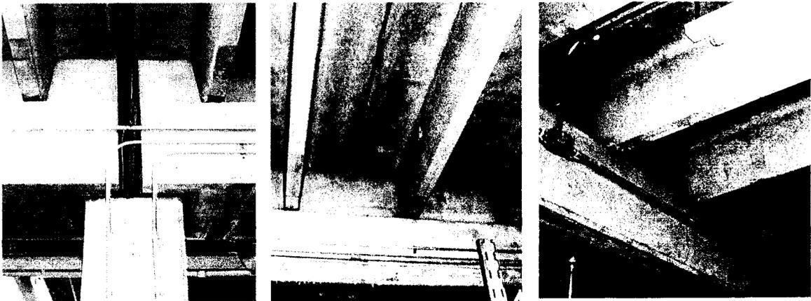
**Figure 2-9: Interior framing and connections between the precast elements.**
