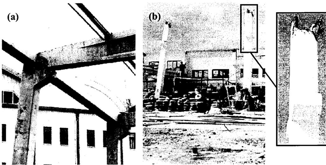
Figure 1-5: Member distress at the roof level: (a) pounding of precast elements (Posada & Wood, 2002); (b) inadequate beam-to-column connections (Saatcioglu et al., 2001).
