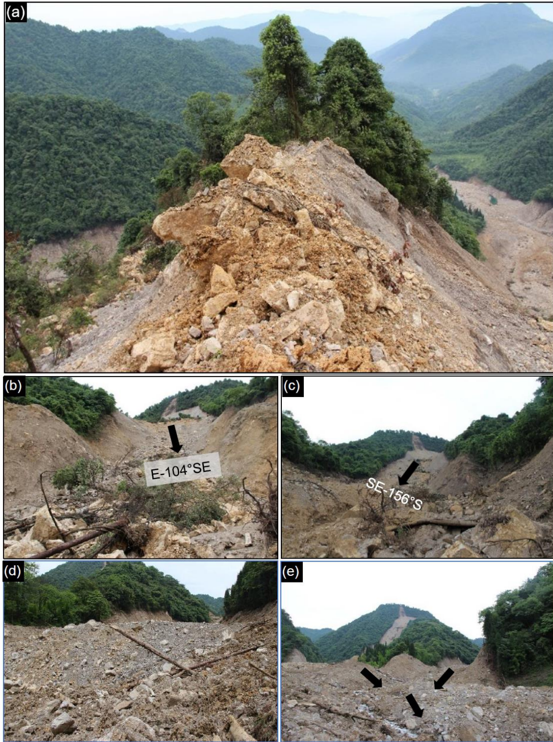
Figure 4 - 4. Characteristics of the Tangjia Valley rock avalanche: (a) the mountain ridge controls the landslide initiation; (b) The upper part of the Chunjianwo valley towards the source area; (c) The upper part of the Gangoutou valley towards the source area; (d) Deposits in the Chunjianwo Valley; (e) The two streams converge into the Tangjia Valley.
