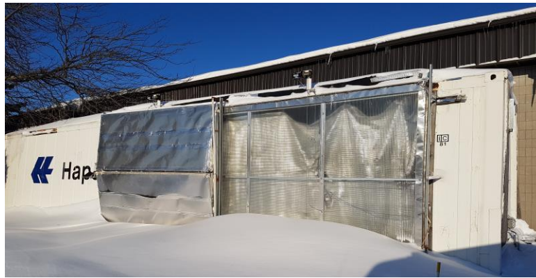
Figure 2.1 Outside of the CING, December 2017
