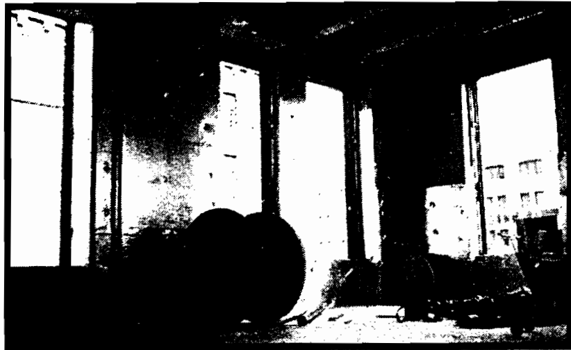
Figure 7.18 Insulation fixed on inside face of exterior masonry wall
