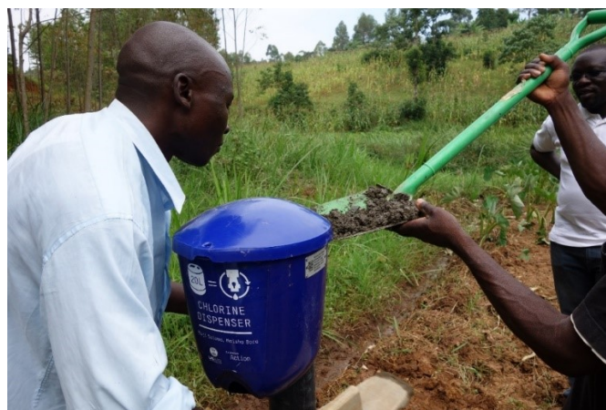
Figure 10: Installing a new dispenser in Ninoto (Photo by Fiona Gedeon Achi)
