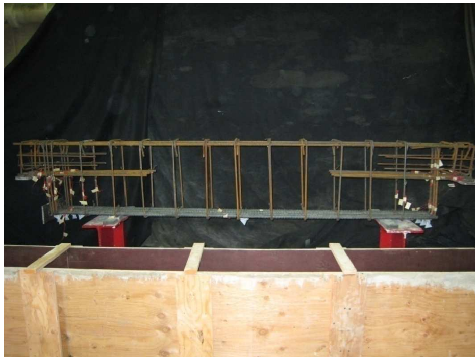
Figure 2.20 Overall view of reinforcement cage of DB2
