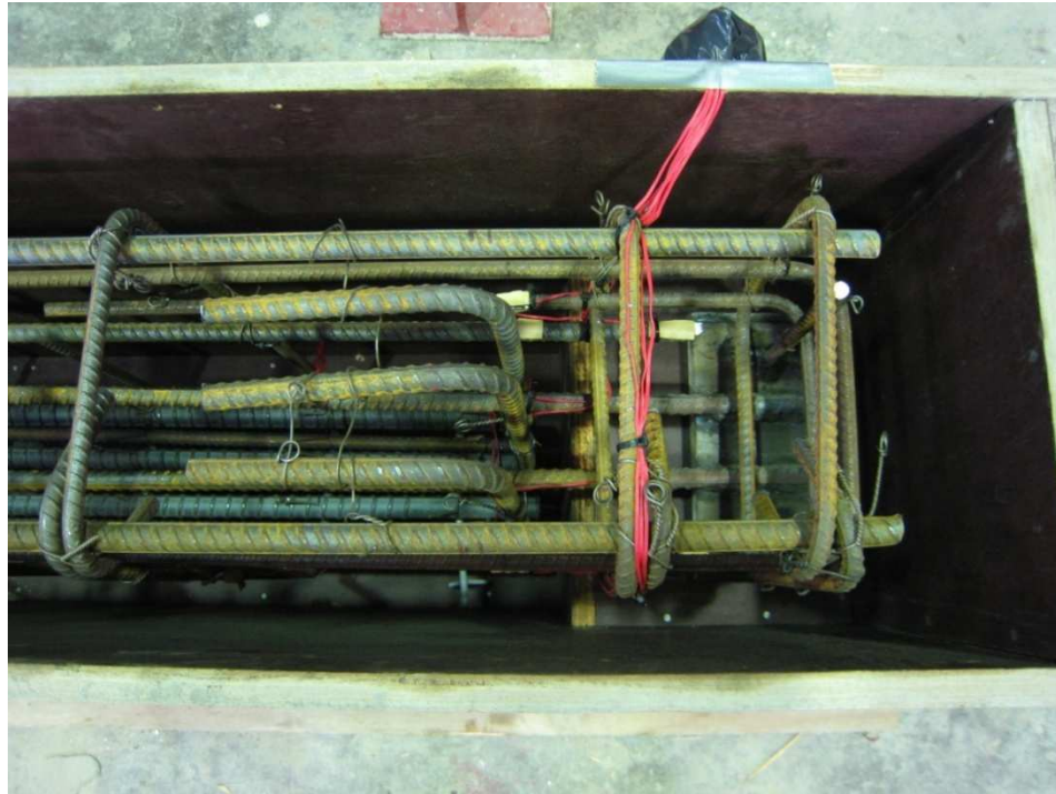
Figure 2.25 Reinforcement cage in formwork at dapped end of DB2-S
