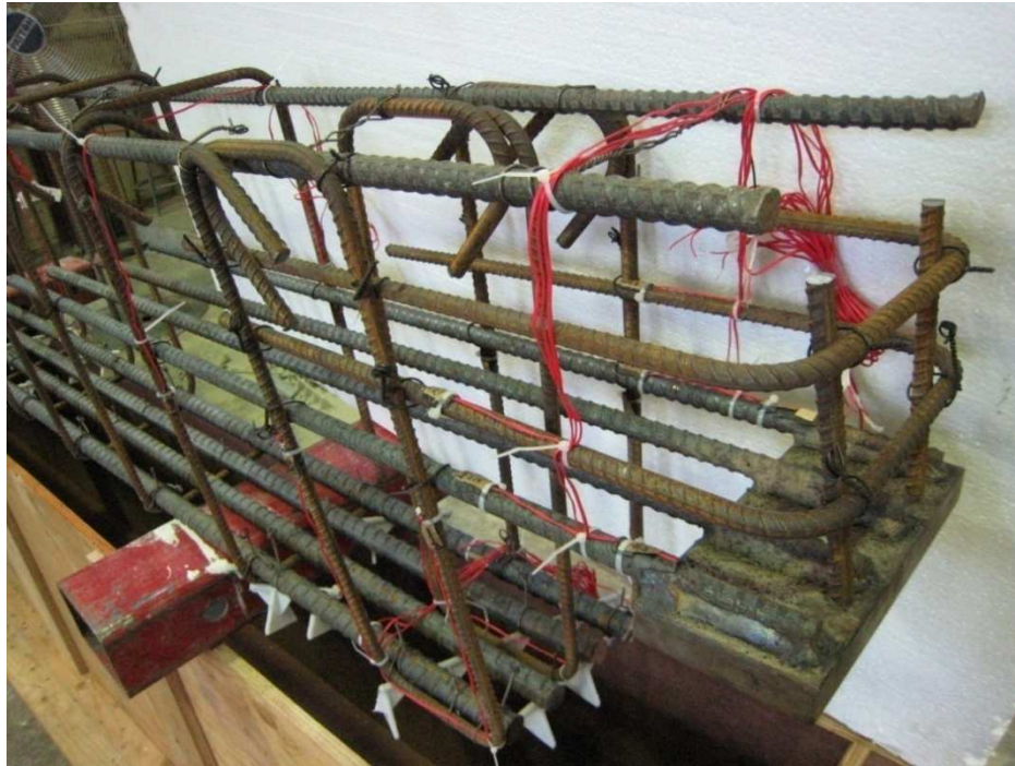
Figure 2.19 Reinforcement cage end view at north side dapped end of DB1
