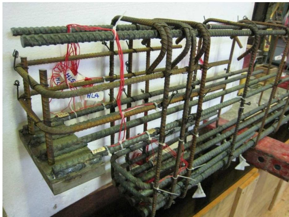
Figure 2.18 Reinforcement cage end view at north side dapped end of DB1
