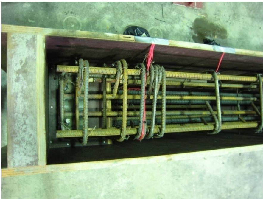
Figure 2.24 Reinforcement cage in formwork at north side of dapped end of DB2
