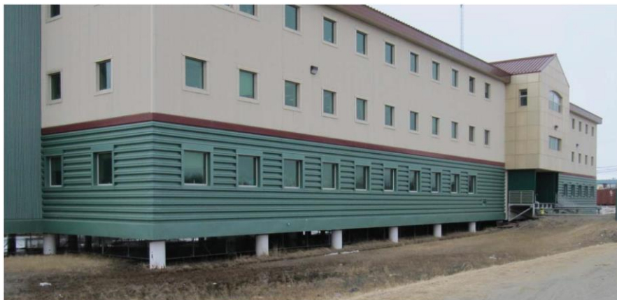
Figure 2.8 Example of open ventilated crawl space under heated building (Perreault, 2016)
