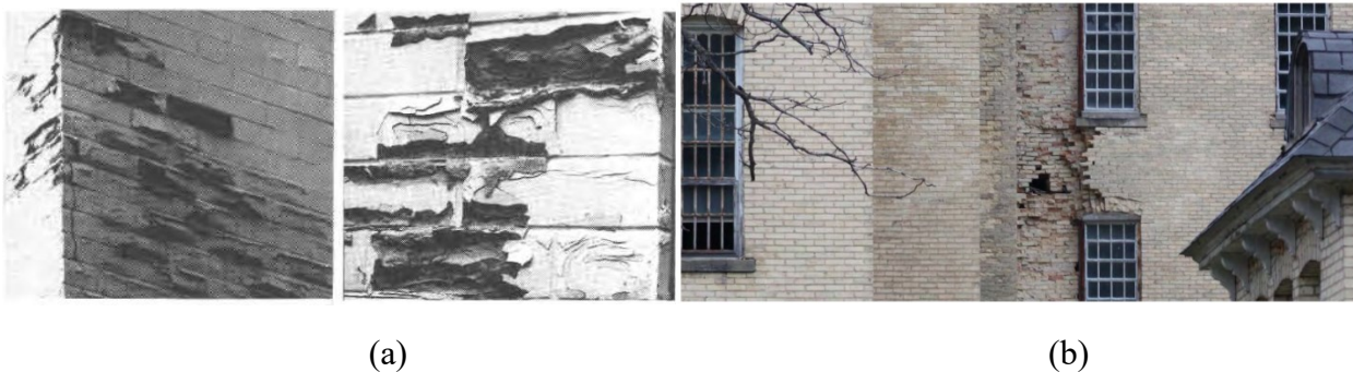
Figure 1.5. (a) Brick spalling caused by freezing and thawing (Maurenbrecher & Suter, 1989); (b) Severe freeze-thaw damage caused by local moisture accumulation (Trainor, 2019)
