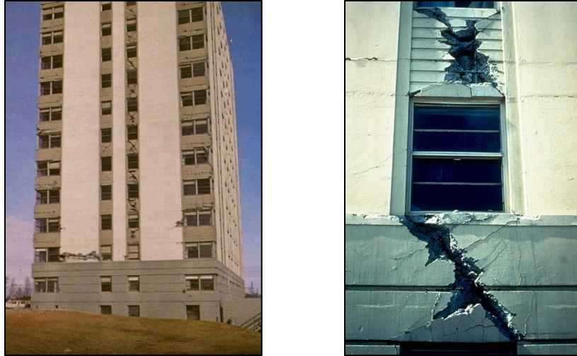
Figures 1.5 – Characteristic failure of short coupling beams during the 1964 Alaskan Earthquake (Hansen et al., 1966 and Faison et al., 2004)
