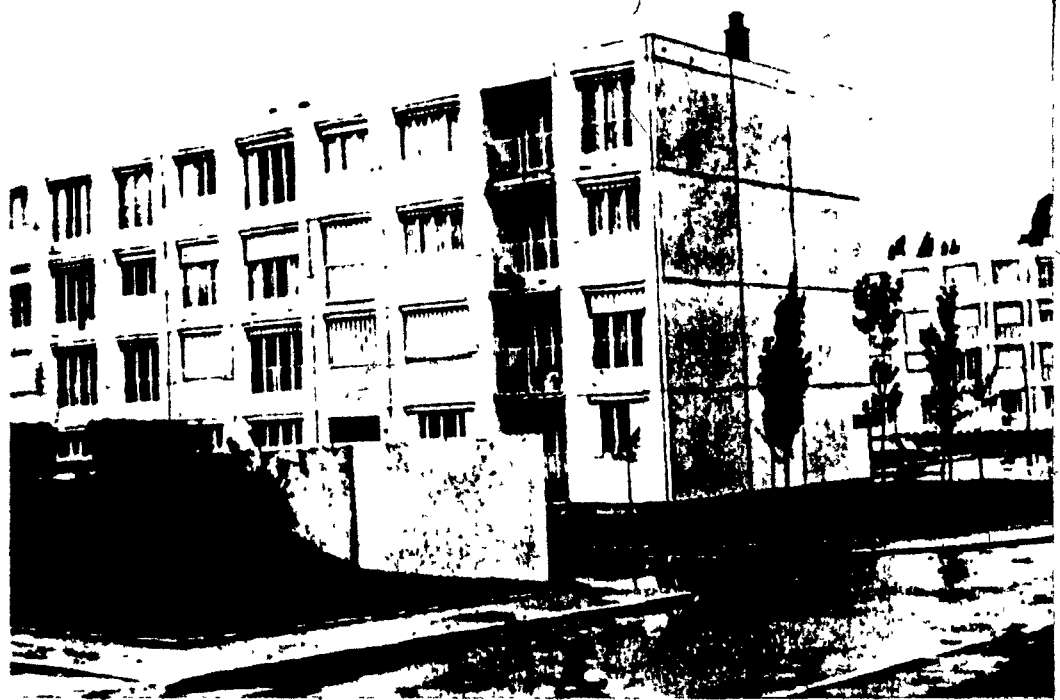
medium rent apartment project
