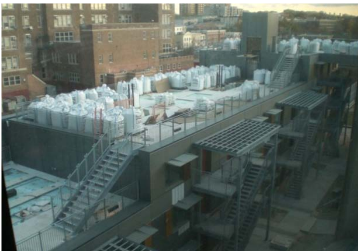
Figure 3.47: Construction of terraced green roof garden before application of base soil.
