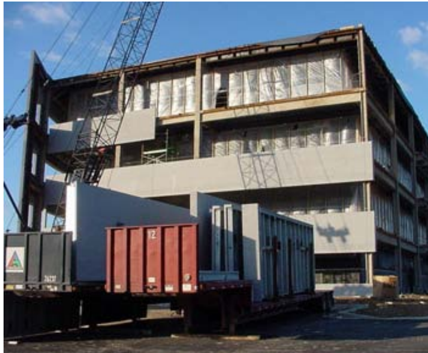
Figure 2.15: Image of panelization design method during construction (Source: http://www.slenderwall.com/panelization.shtml , 2012).
