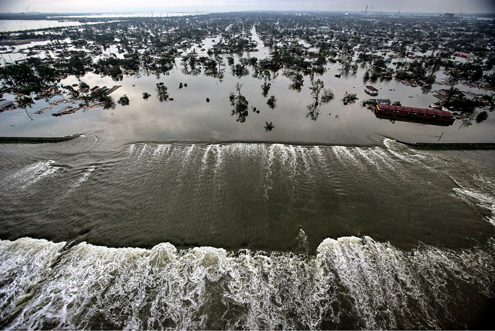
Figure 9. Water pours into New Orleans' Lower Ninth Ward through a breached levee along the Industrial Canal on 30 August 2005. Source: Reuters
