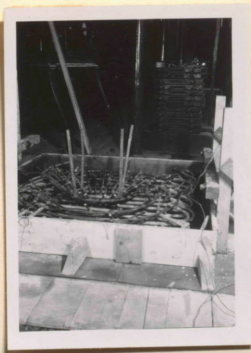
Fig. 23 Reinforcement for slab J
