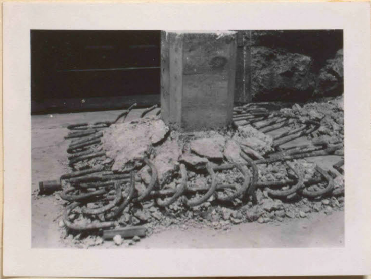
Fig. 20 Slab G - broken up
