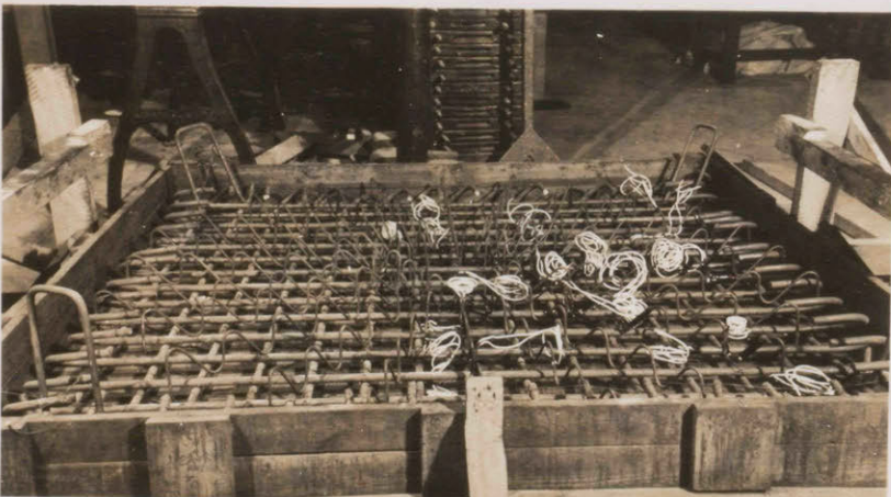
Fig. C: Gersovitz N - shaped reinforcement
