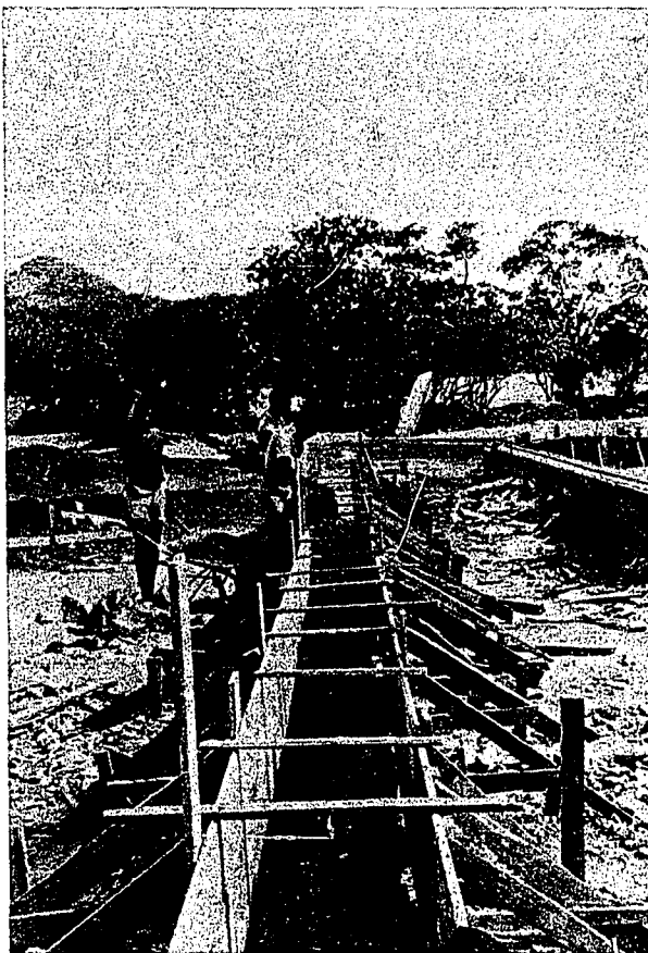
Plate No. C-3 indicates the construction of a concrete rail of a solar still bay.
