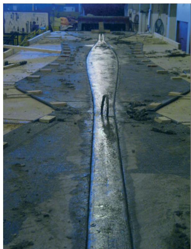
fig. 5 Beam model formwork and full-scale fabric formwork beam cast, Mark West, 2003
