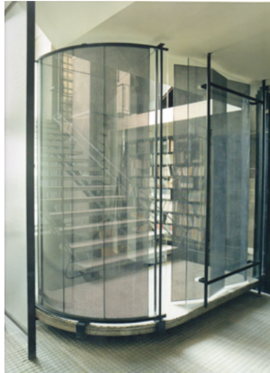
Fig. 5.12 Mechanical screen and stair landing, Maison de Verre
