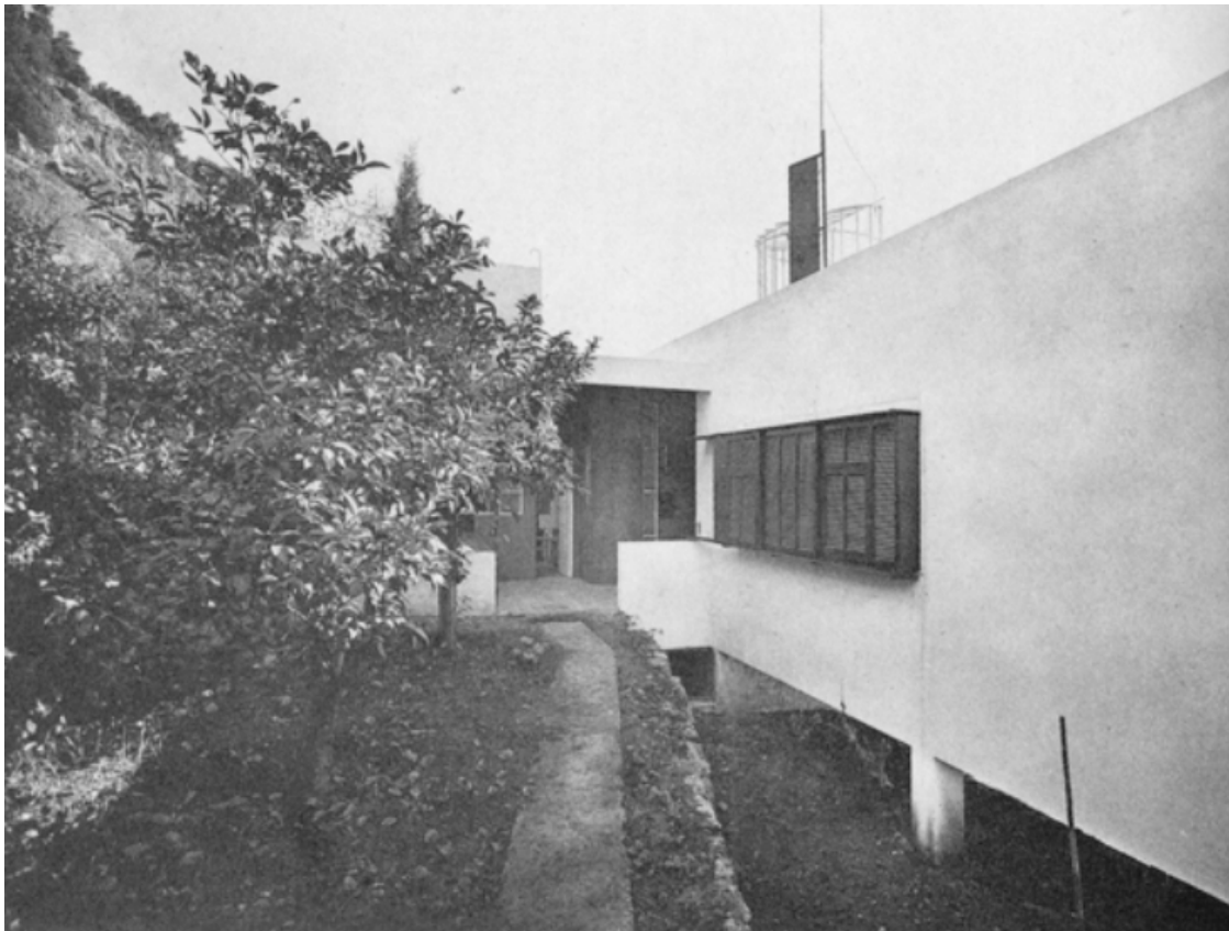
Fig. 5.26 Approach to E.1027
