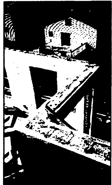
Figure 4.5: Permanent insulated formwork / concrete system. Source: courtesy of Polycrete, 1998.
