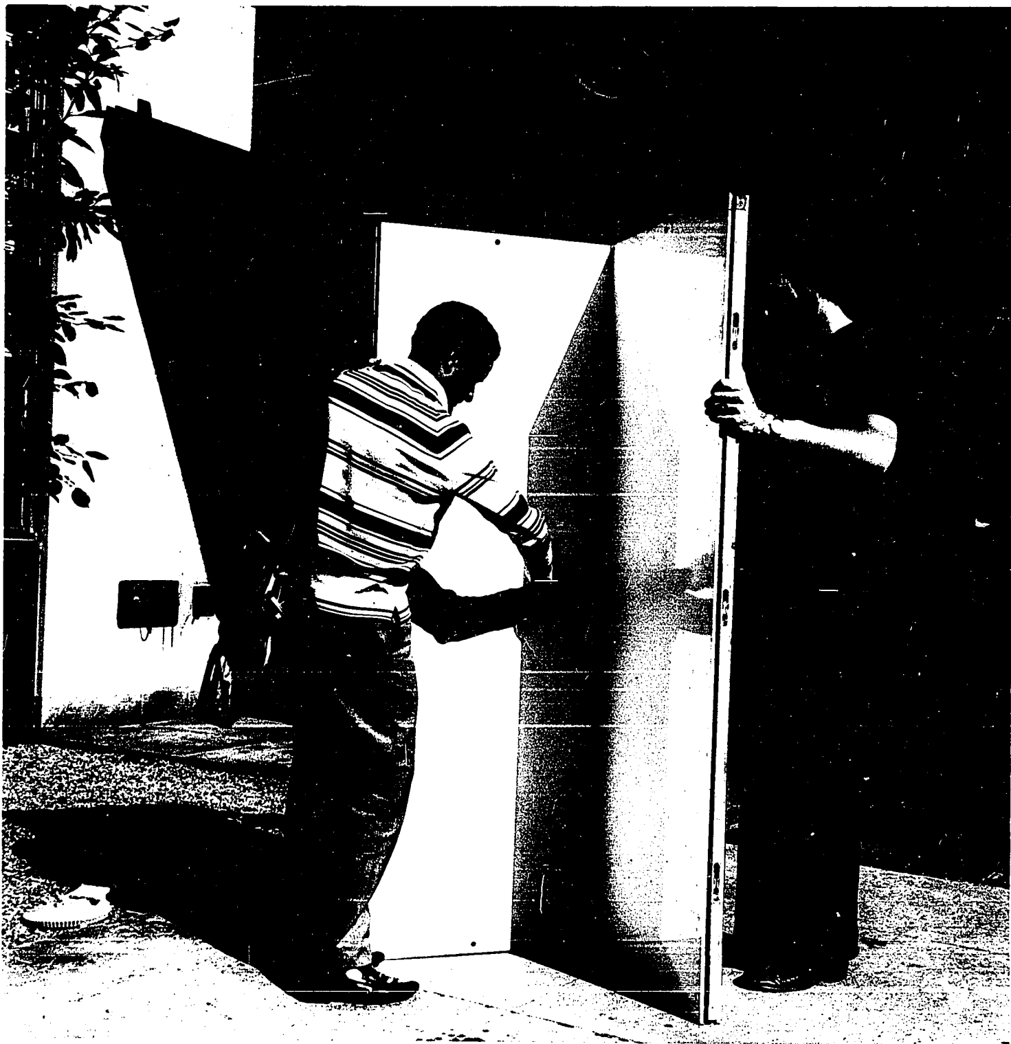
Above, the assembly of two panels to form a meeting of ninety degrees.
