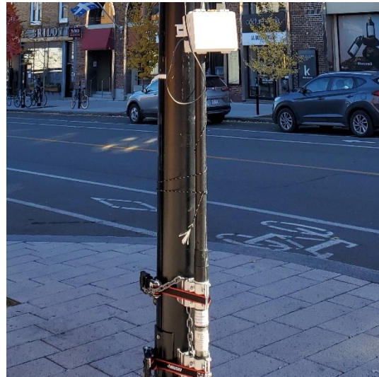
b- Processing unit and battery box installation
