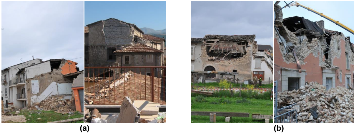
Figure 3 Typical OOP failure mechanisms in the 2009 L'Aquila earthquake with collapses of (a) gables and (b) main façades.
