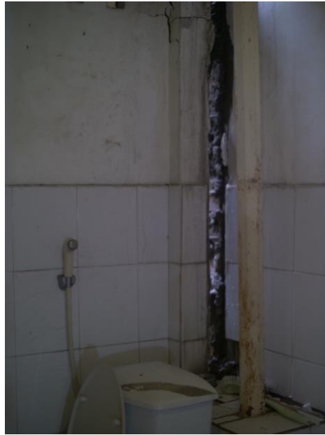
Figure 7.9 Cracks in Mr. Ong's bathroom. Source: Author
