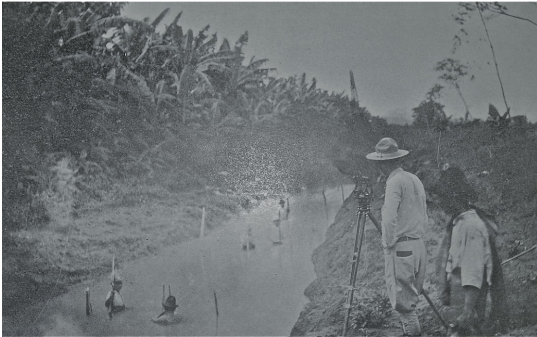
Surveying party occupied in direction drainage ditch construction – United Fruit Company Medical Reports v.18, 1929.
