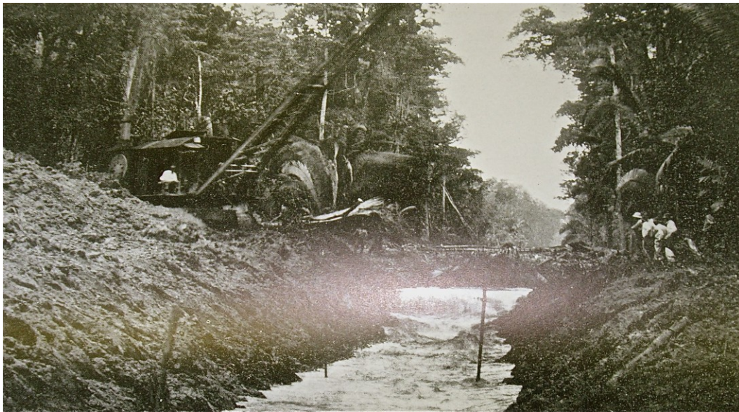
Mechanical dragline digs drainage canal – United Fruit Company Medical Reports v.18, 1929.
