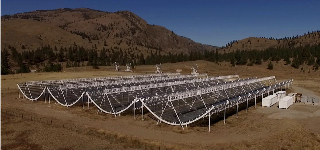
**Figure 2.1:** A photograph of CHIME as taken on 15 September 2016 in Penticton, British Columbia. The four N-S cylinders are visible along with the focal lines containing the 256 dual polarization feeds. Image courtesy of CHIME/FRB Collaboration (2018) [1].
