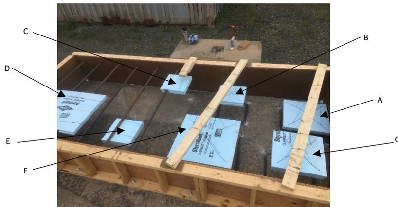
Figure 3-2. Concrete formwork and artificial delamination in the plate. (Photo courtesy: Institut de recherche d'Hydro-Québec, Canada).
