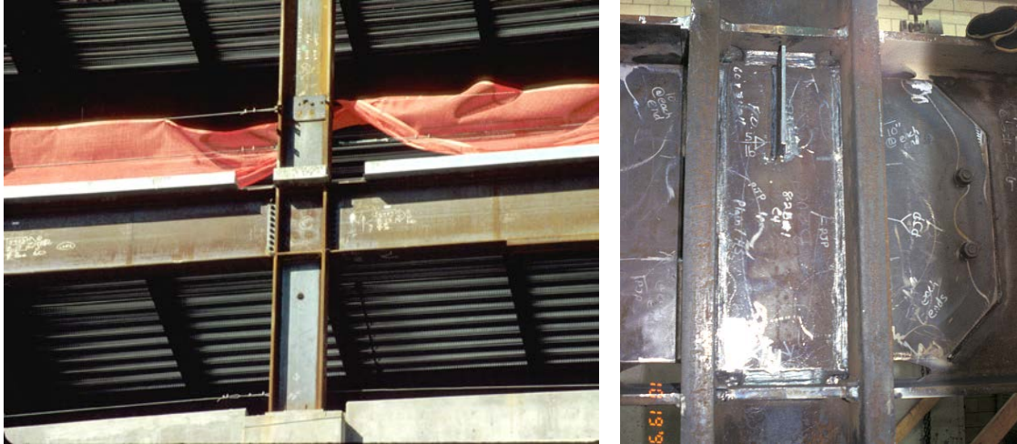
Figure 1.2: Real life examples of prequalified connections with doubler plates (courtesy of Prof. M. Engelhardt, University of Texas Austin)
