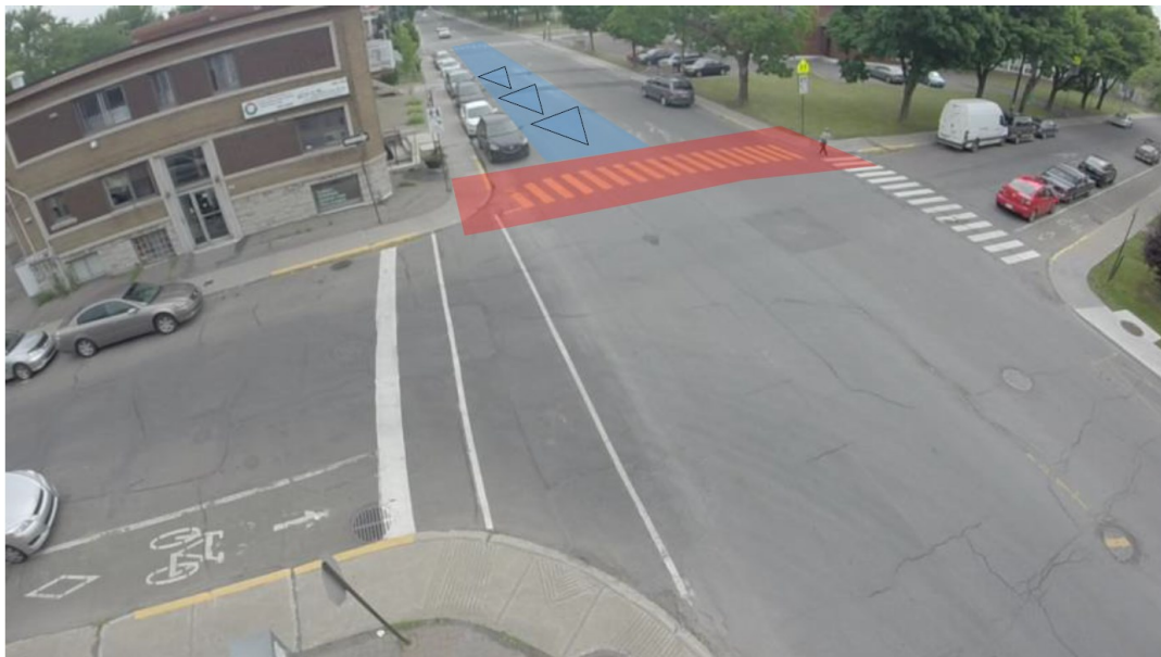
d) Site B-4 Beaubien-27e: Crosswalk located at the intersection of Rue Beaubien and Avenue 27e. The crosswalk crossing is on Rue Beaubien, a two-ways and one lane street per direction.
