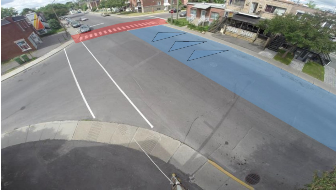
e) Site Z-5 13e_Belair: Intersection controlled with stop signs in all the approaches at Avenue 13e and Rue Bélair. The crosswalk is on Rue Bélair, a two-ways and one-lane street.
