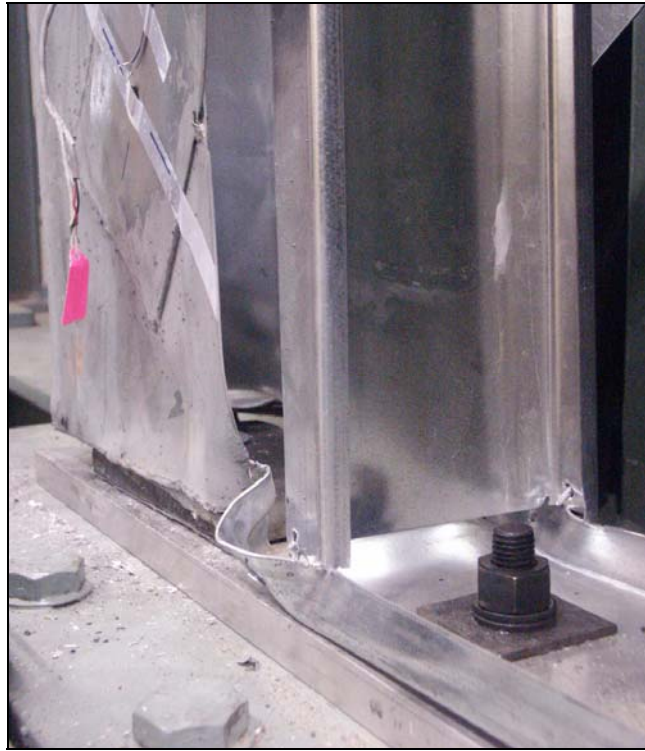
Figure 46: Punching shear failure of the track and screw pull out failure between the interior stud and track in specimen 6B-C
