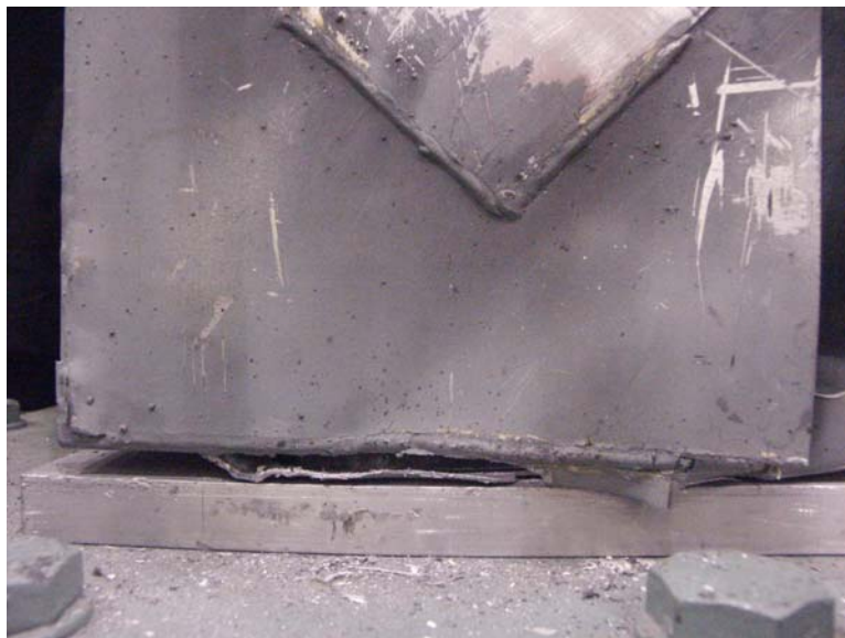
Figure 98: Punching / shear failure of bottom track : Specimen 4B-C
