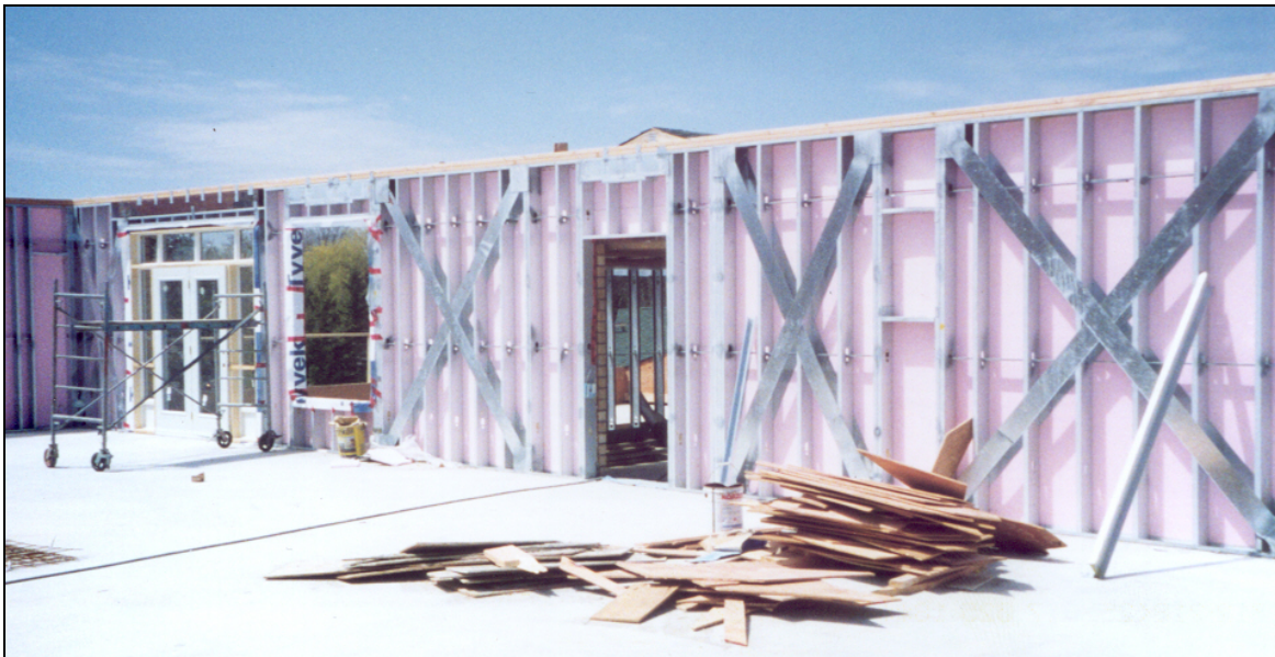
Figure 1: Strap braced walls under construction
