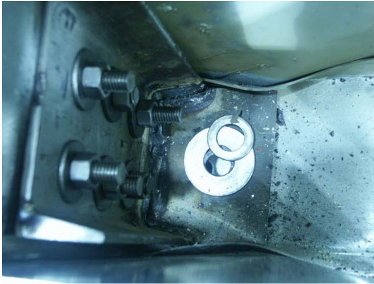
Figure 105: Anchor rod failure : Specimen 5C-M
