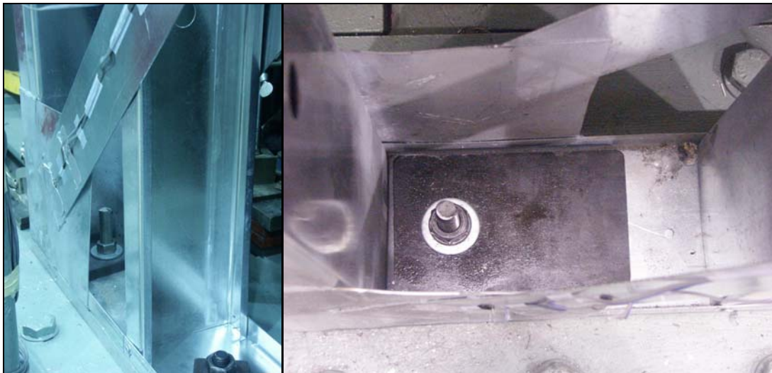
Figure 12: 101 mm (4'') strap brace connection and holddown detail prior to testing
