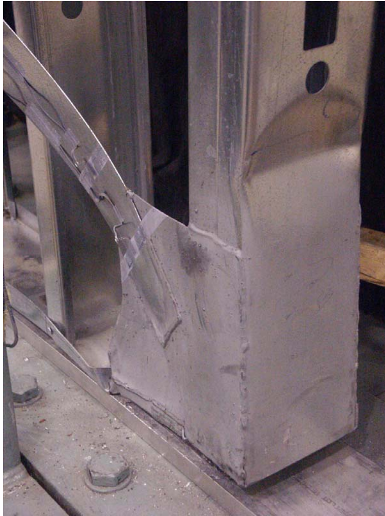
Figure 97: Local buckling of chord studs : Specimen 4B-C
