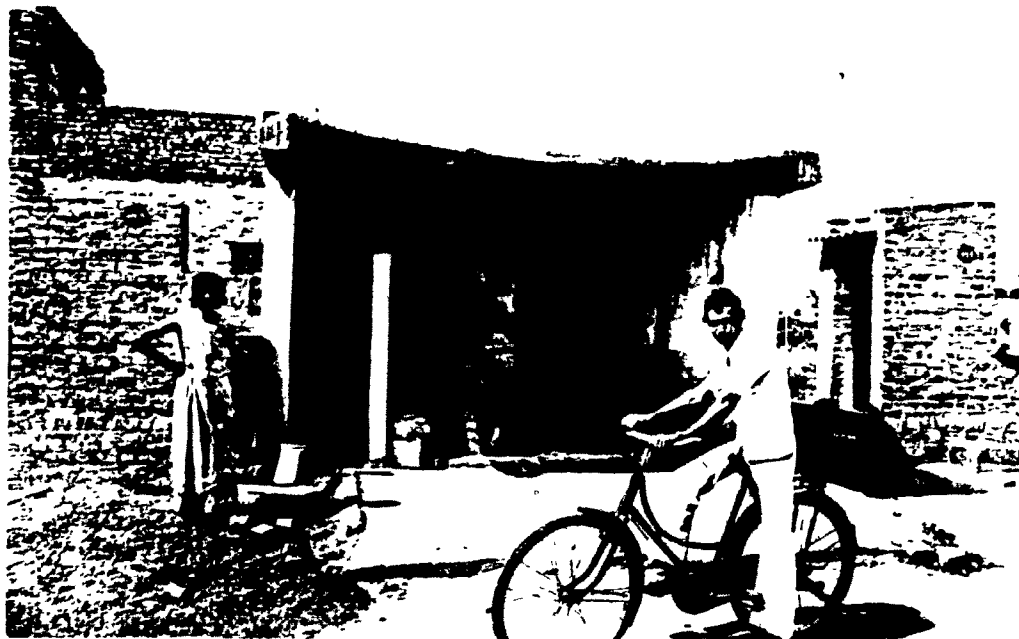
Unsuccessful roof slab construction by owner. A brick pier was added to support the slab after this photo was taken.
