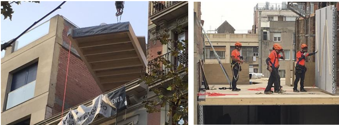
Figure 3.26 Left: Location of Novadomus' prefabricated slabs. Right: View of the walls being installed. Source LCT (Enric Granados 69, Clase Energética A, 2015)
