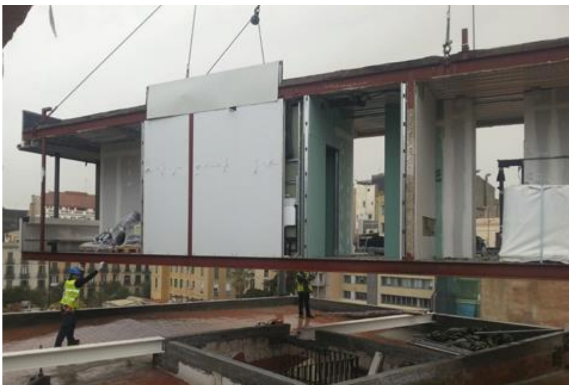
Figure 3.54 Picture of the central structural intervention on Aragó 359: the chained forged beam is seen at the bottom of the picture. Source: LCT Website (Aragó 359 y Roger de Llúria 41, 2015)
