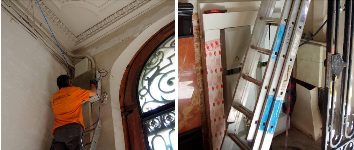
Figure 3.12 Left old electric box. Right: Updated set of boxes with a higher electric capacity. Pictures taken at Aragó 277. May 29, 2018
