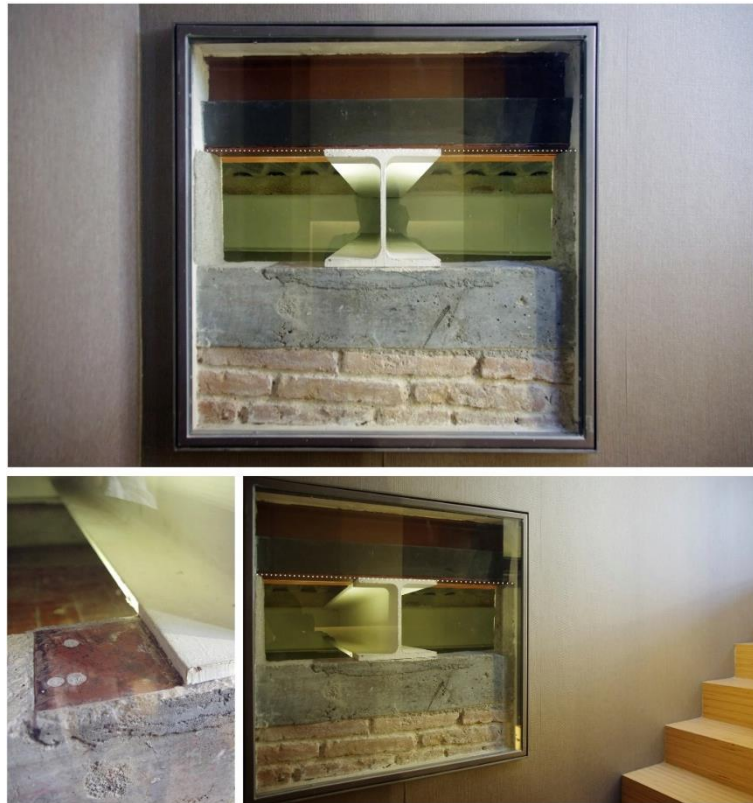
Figure 3.7 Images of the anchoring system at the rooftop expansion Roger Lluria 41 (LCT central office). The brick wall at the bottom is the old bearing wall; then, a chained concrete beam which is merged with transversal steel beams screwed. These two level and support the modules that sit above it as it can be seen in the black and red structure. May 29, 2018.
