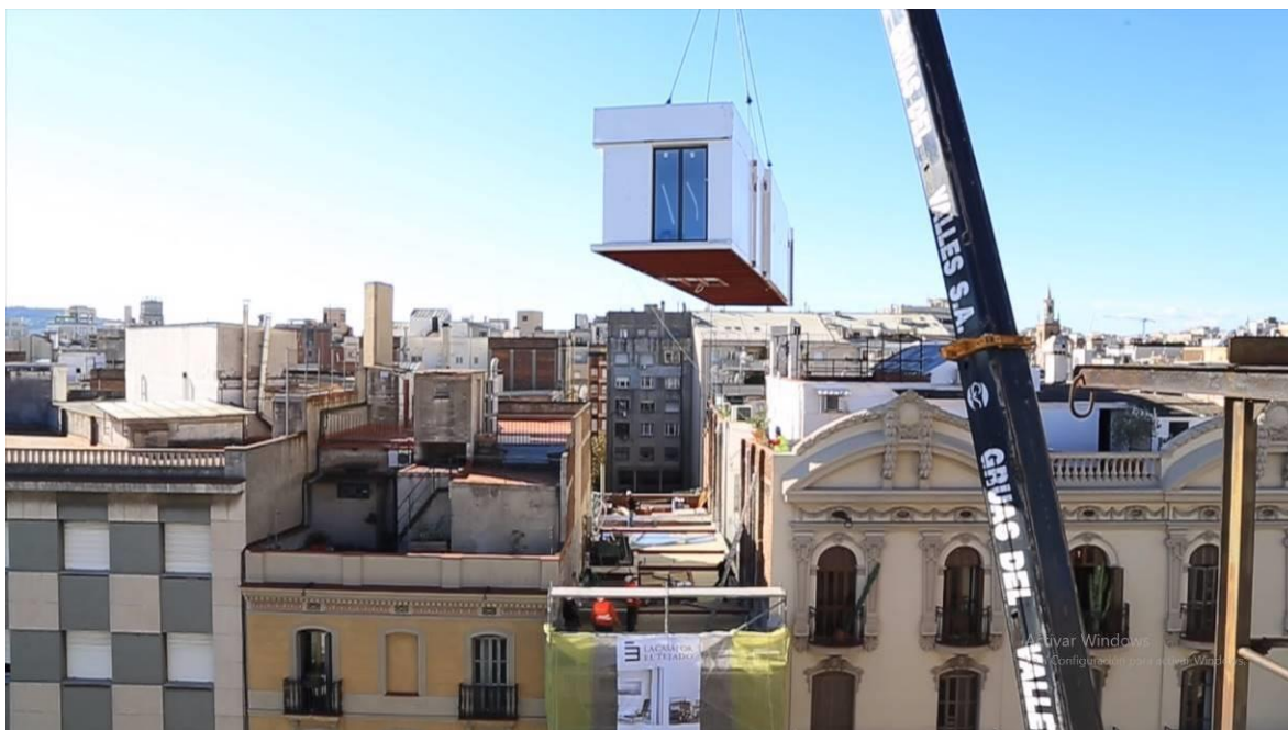
Figure 3.65 Installation of the largest module at Girona 81. Adapted by the author from the video by Artes. (Girona 81, 2014)
