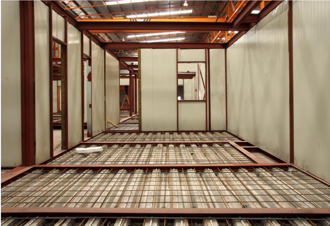
Figure 4.11 Standard module. Uses a 3D steel structure with steel deck and forget cement for flooring and roof. The envelope is built using a drywall system that consists of a sandwich panel and gypsum board. Gava factory June 6, 2018.
