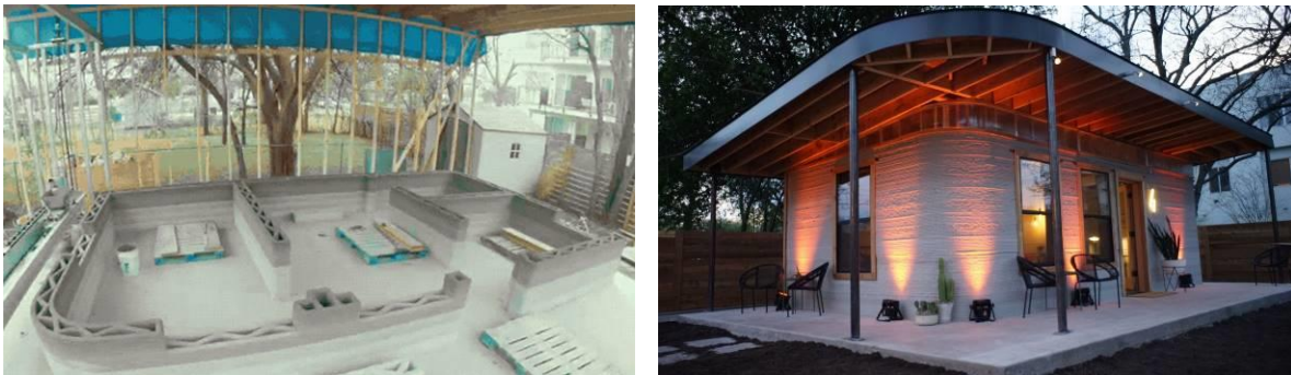
Figure 4.16 Left: Layering of the cement walls using a 3D printer by New Story. Right: Same house finished. Source: Rob Reuland, Designboom website, “3D-print a home in 24 hours, a game changer for global homelessness” March 18, 2018
