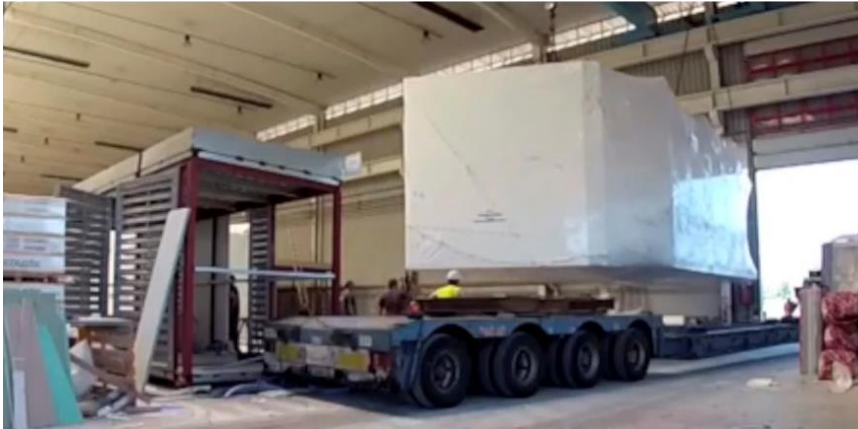
Figure 4.5 After three months, the prefabrication phase is done. All the modules need to be shipped to the designated location to go into the post-installation work. Source: Dirksen (Popout prefab flats assembled and stacked on Barcelona roofs, 2015)
