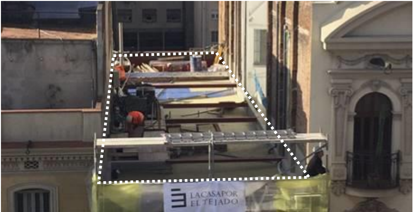
Figure 3.64 View of the rooftop preparation with the chained beam on top of the support walls and the transversal steel beams. In this case, the rooftop also received a waterproofing treatment to protect the existent penthouse from infiltrations while the new unit arrived. Source: LCT Website (Girona 81, en una Mañana, 2015)
