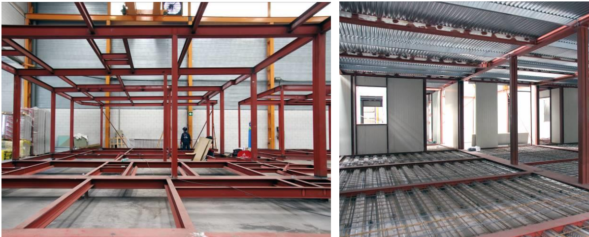
Figure 4.4 Left: Picture of new modules at Gava, LCT's prefabrication facility. Right: Picture of modules with the exterior panels and steel deck already in place, same location. June 6, 2018
