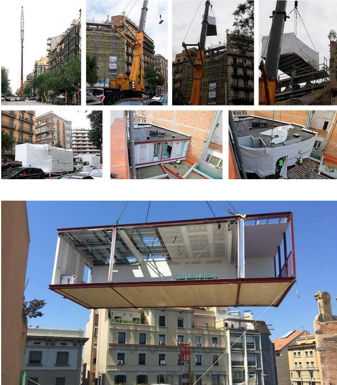
Figure 3.41 Images of the process of transportation and installation of Letamendi 29's prefabricated modules. Source: LCT & Perea, Rafael (Áticos Nuevos en Finca Antiguas, 2014)
