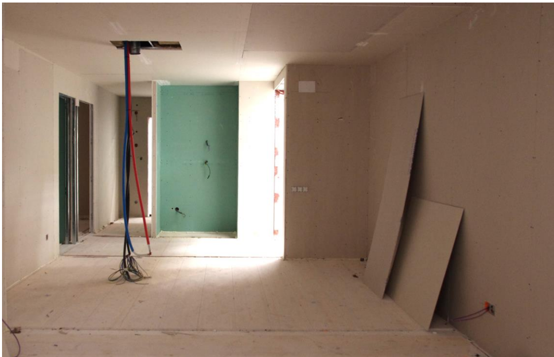
Figure 4.11 Standard module. Uses a 3D steel structure with steel deck and forget cement for flooring and roof. The envelope is built using a drywall system that consists of a sandwich panel and gypsum board. Gava factory June 6, 2018.
