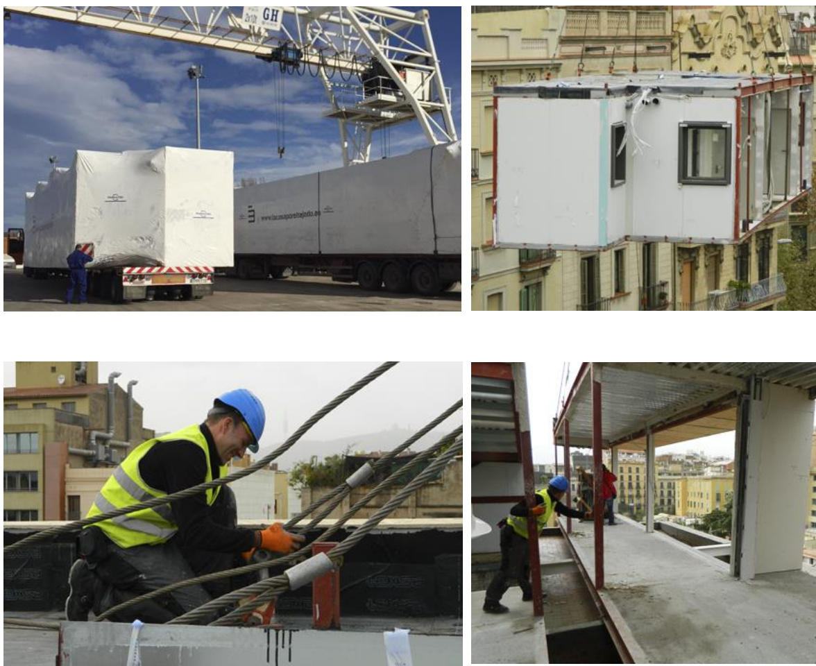
Figure 3.51 Pictures of the process of transportation and installation of Aragó 359's prefabricated modules. Source: LCT Website (Aragó 359 y Roger de Llúria 41, 2015)
