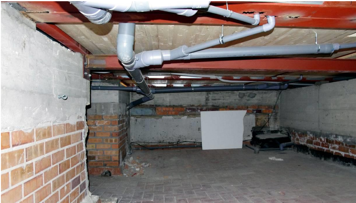
Figure 3.11 View from the air chamber between the new modules at Aragó 277 and the existent building. It illustrates the hydraulic network that comes from the modules and goes to the Patilejo on the far left. May 30, 2018.
