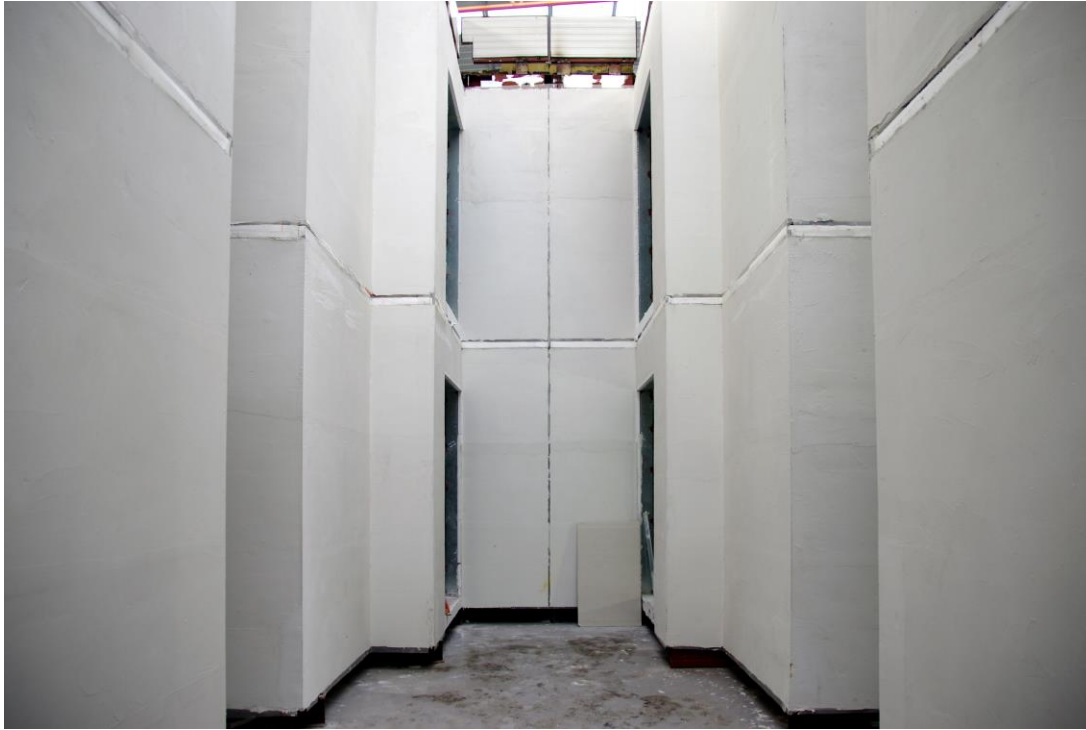
Figure 4.13 This picture clearly illustrates the combination of different modules in a single project. The group of modules on the bottom uses the system expressed in Figure 4.11 and the ones on the top use the one described in 4.12. Gava factory June, 6 2018
