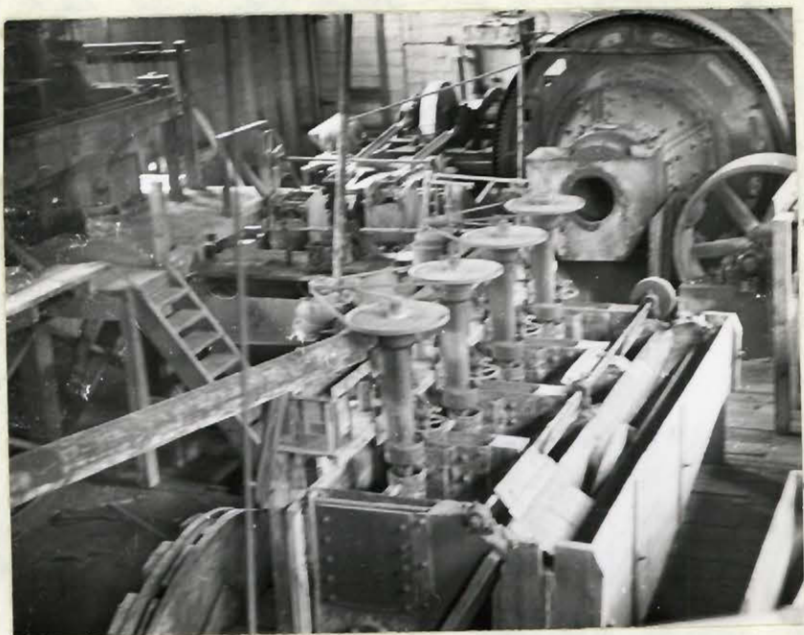
Plate XL: Interior of mill, Jardun Mines, showing flotation cell bank.
