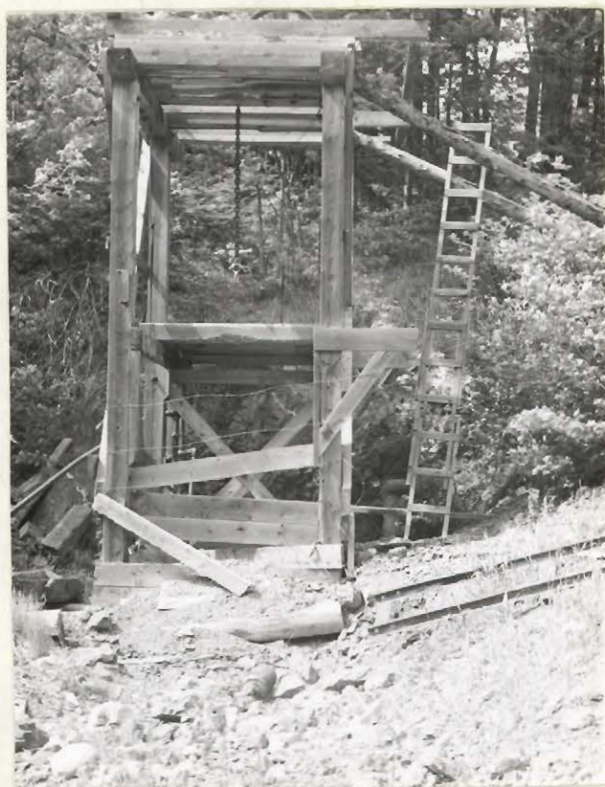
Plate XXXVII: Headframe above original workings of the Victoria No. 1 vein, Jardun Mines.
