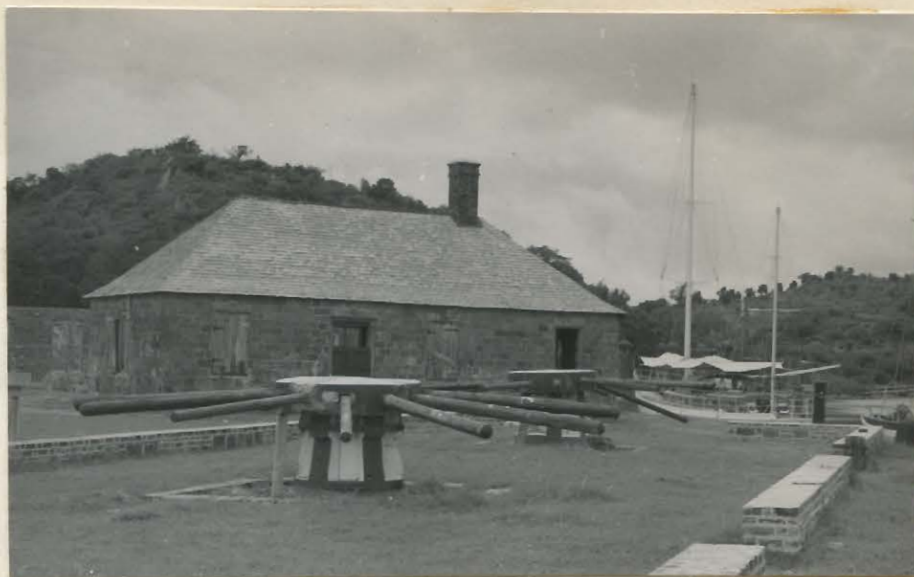
Fig. 51.--Capstans at English Harbour. These were used to careen the Royal Navy's warships before the age of steam. In the background is the galley.
