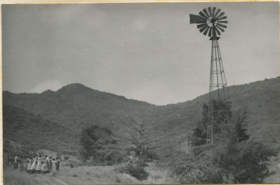
Fig. 44.--Well at Cade Bay. The alluvial deposits of the valleys cutting into the volcanic district provide good sources for water. This well was erected during the last war. In the photo some workers are receiving weekly wages.
