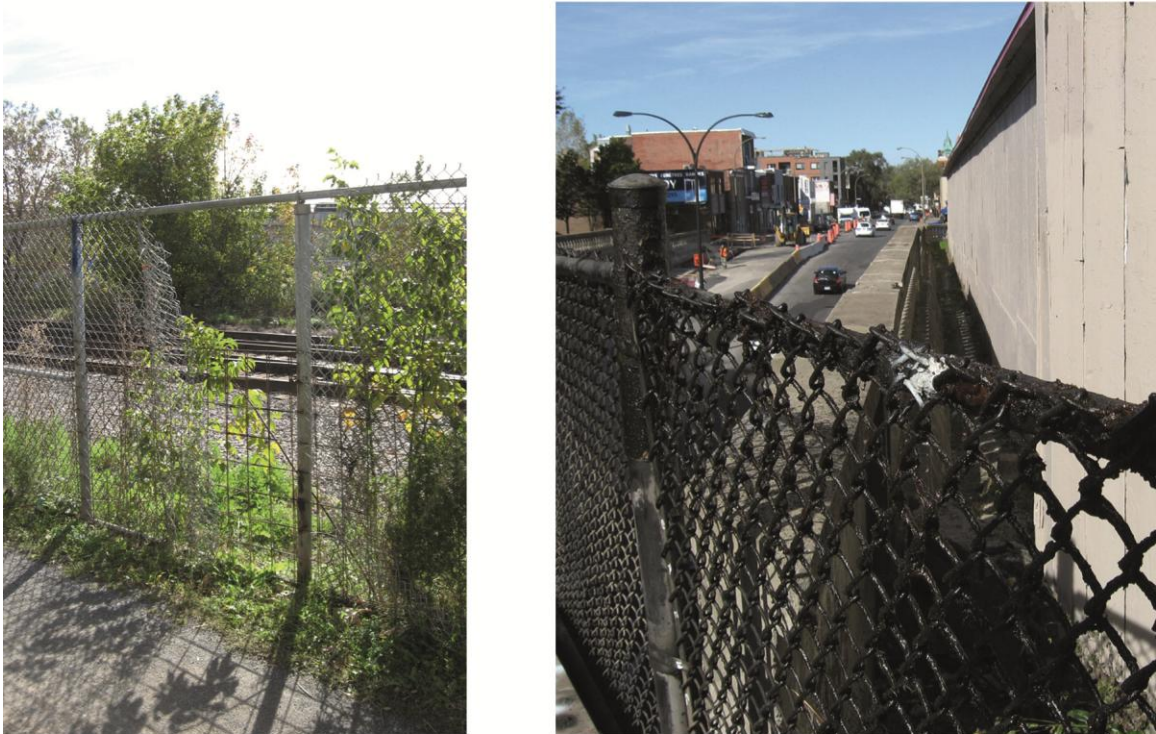
Figure 3.20: The battle for permeability on the railway of the Bellechasse site. On the left, a part of the fence that has been damaged, fixed with reinforcement and damaged again. On the right, the fences are covered with grease in order to prevent passers-by from taking a short cut.
