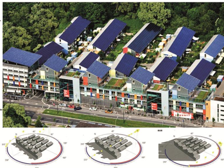
Figure 2.3: Freiburg, Germany. Solar power and mix use. The solar diagrams of the residential complex built on a roof of a commercial building. (Source: rolfdisch.de)
