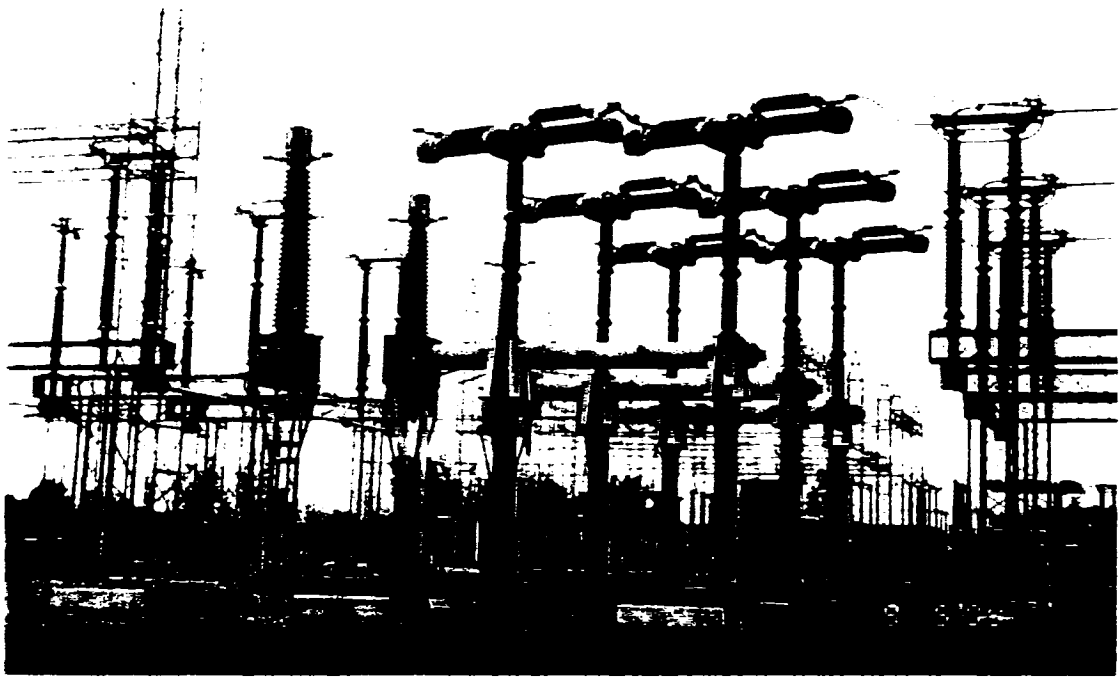
Figure 5.17: Circuit Breaker Delle PK4A with Vulnerable Insulation Supports (Hydro-Quebec, 1999)
