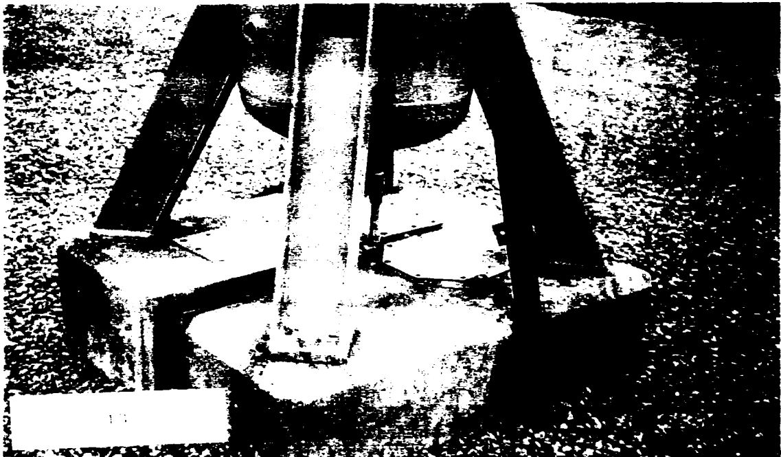
Figure 5.18: Vulnerable Support of Circuit Breaker (Hydro-Quebec, 1999)
