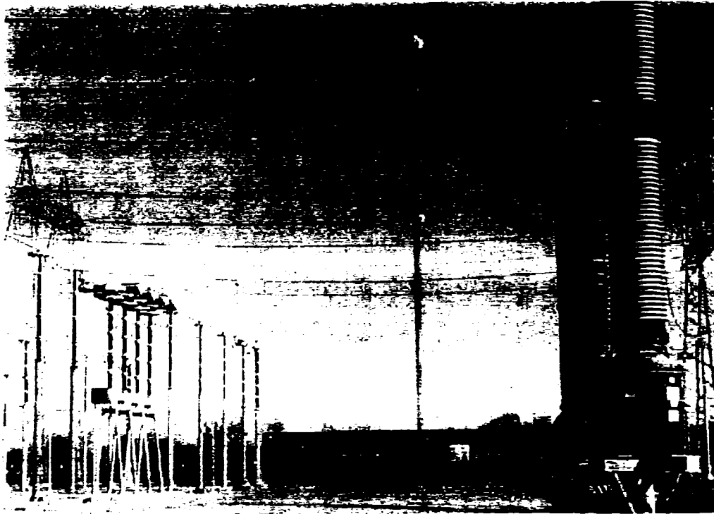
Figure 5.13: PK8C Circuit Breaker with Ceramic and Steel Support (Hydro-Quebec, 2001)
