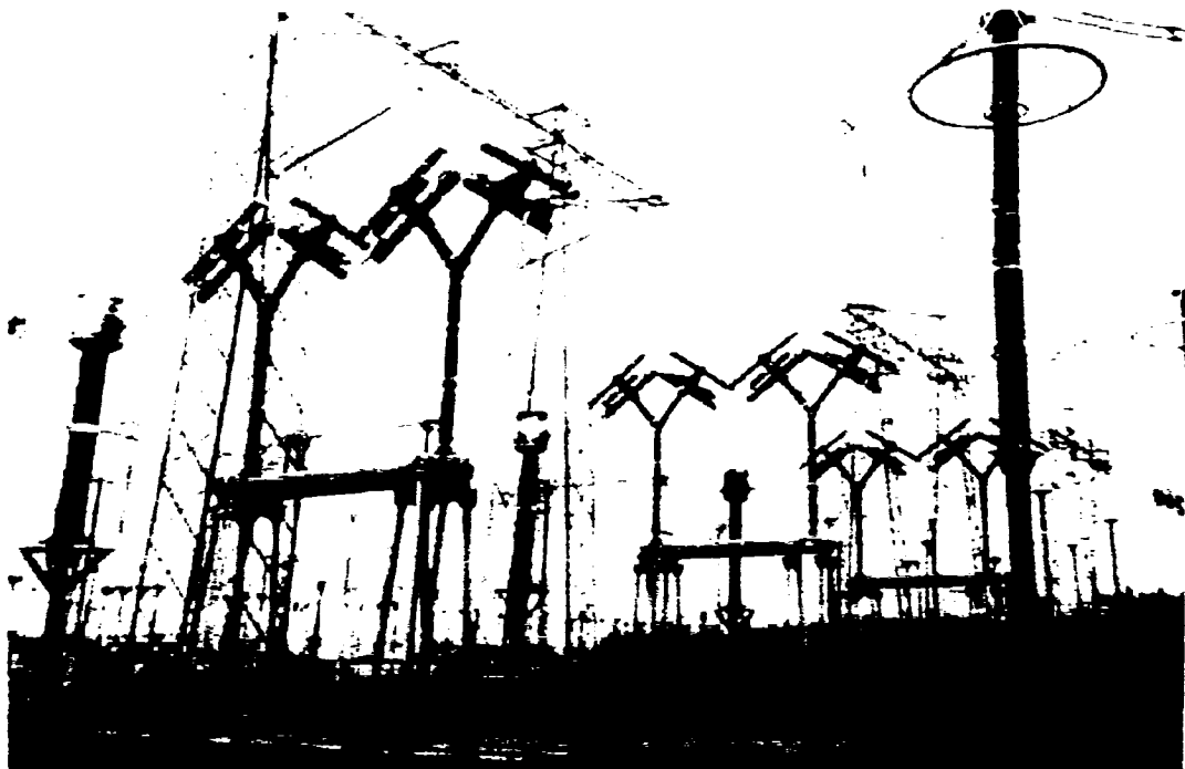
Figure 5.14: Circuit Breaker DLF 735 KV (Hydro-Quebec, 2001)
