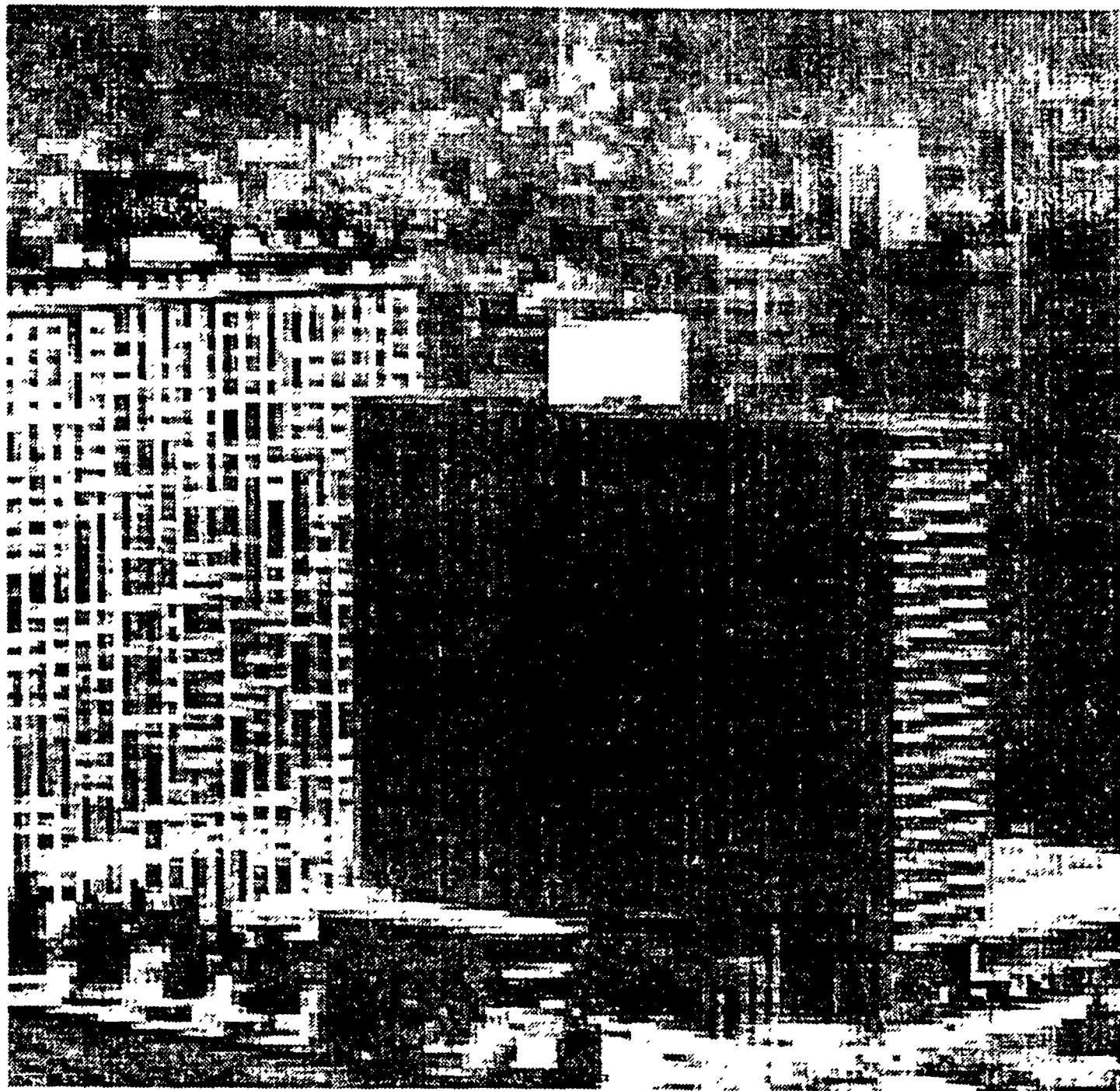
Figure 1.3.a An image of an urban scene 256x256 resolution displayed using dither matrices with 32 effective gray levels. Note that the structure in the left portion of the image contains discernible detail.
