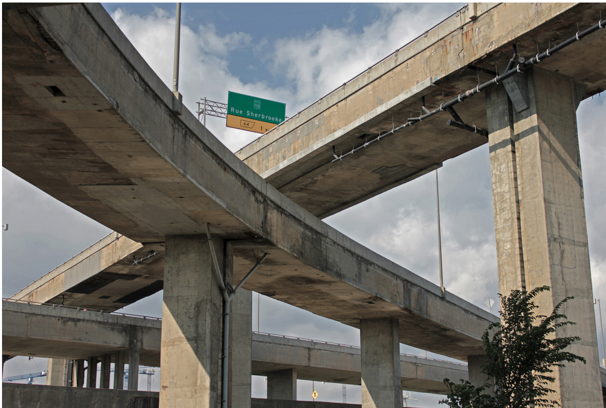
Figure 20: The Turcotte Interchange (mesh reinforcement visible in lower left), 2011. (Photo “Échangeur Turcotte.jpg,” Wikimedia Commons)
