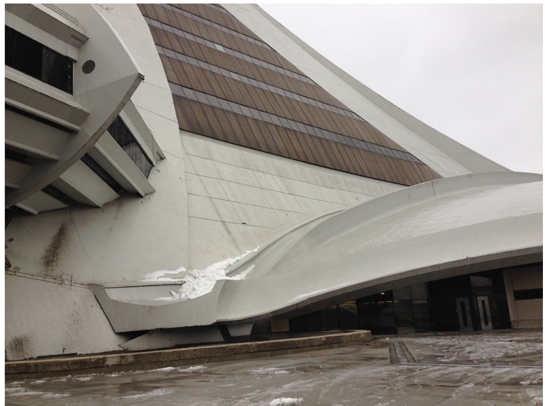
Figures 38 and 39: Photographs showing chipped membrane on roof of the Biôme (left) and the weathering and staining on the base of the Tower (right) (Photos: Author, 2014).
